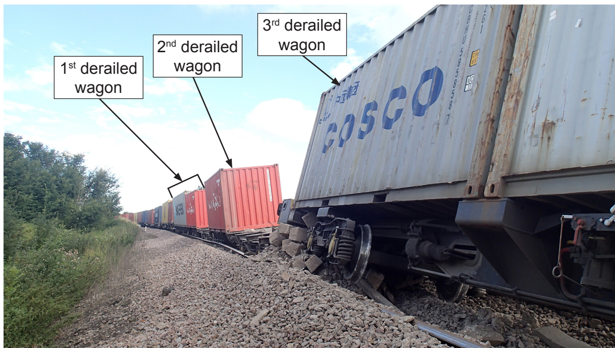
Figure 2: Derailed wagons on site
