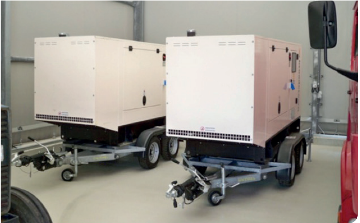
Figure 5: Emergency Diesel Generators at Wylfa
