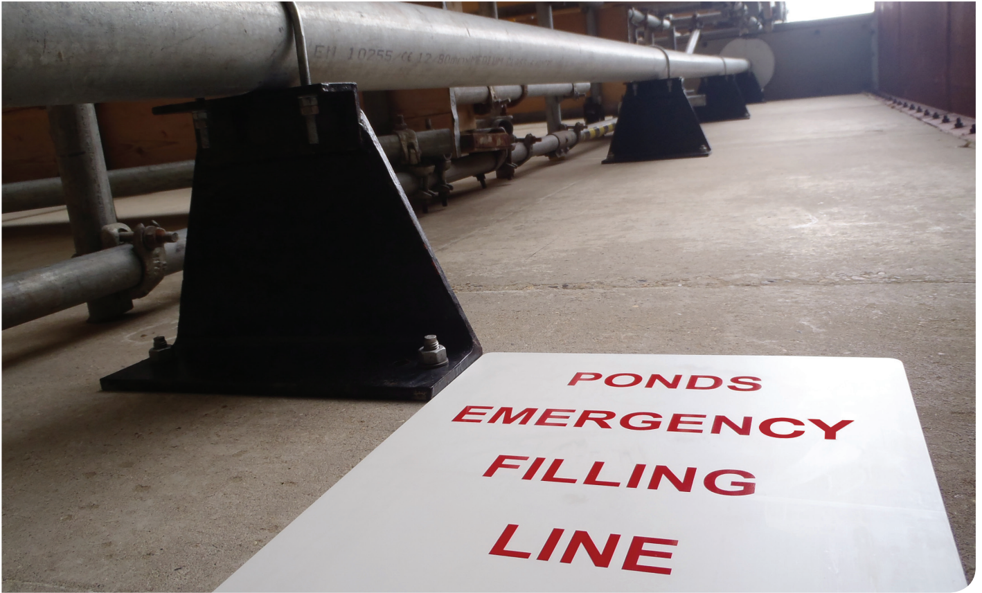
Figure 15: Emergency Spent Fuel Pond Filling Line at Sizewell A
