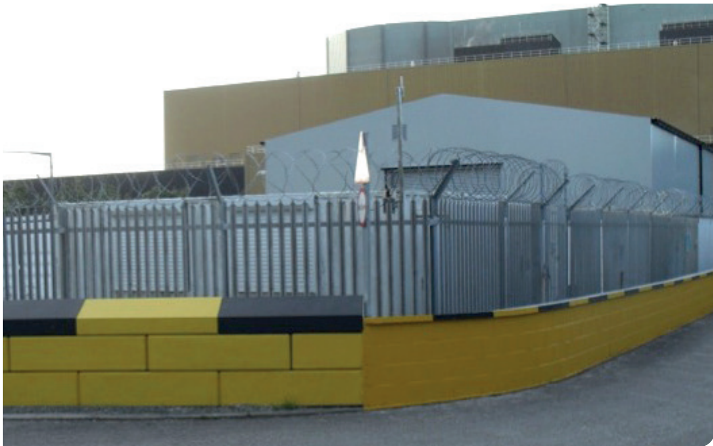
Figure 2: Beyond Design Basis Emergency Equipment Compound at Wylfa
