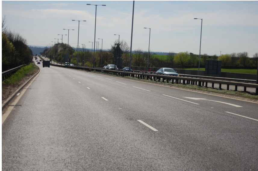
Figure 4.10 – A404 southbound looking away from Handy Cross Junction
