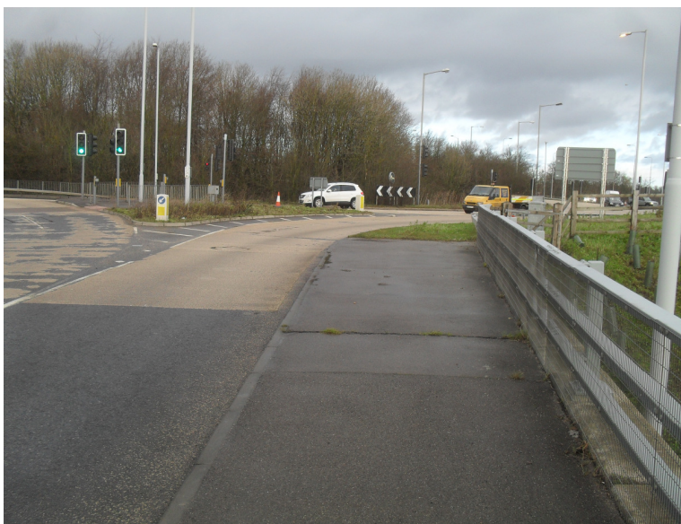
Figure 4.9 – Arm E exit from roundabout (view looking east)
