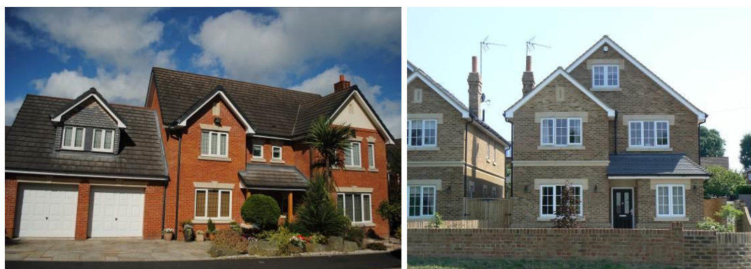
Photo: Two recently-built detached homes. The one of the left has been designed to maximise the use of the available plot.
