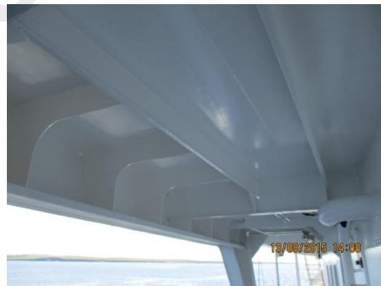
Deck maintenance was exceptional
