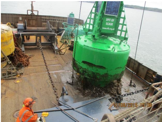
Buoy partly cleaned, scraped of kelp and crustations ready for water blasting
