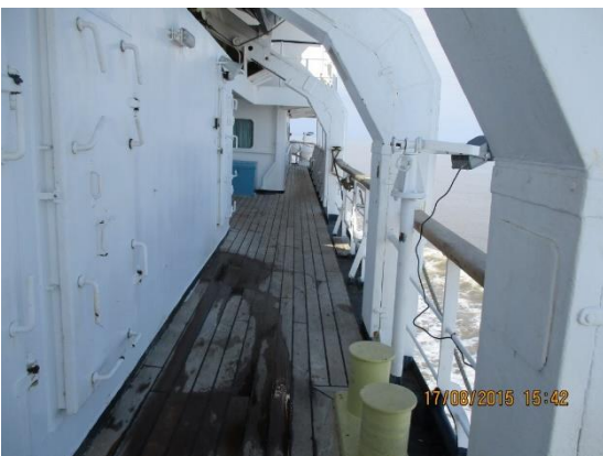
Accommodation decks and accommodation alleyways are well maintained.
