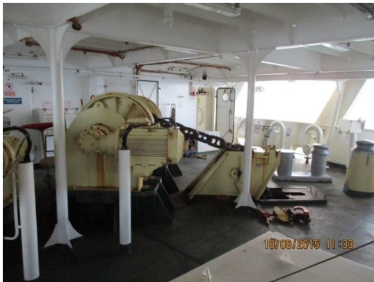
Forecastle area, clean and tidy
