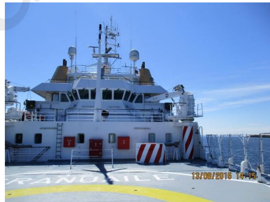
From the helicopter deck looking aft. Maintenance is very good
