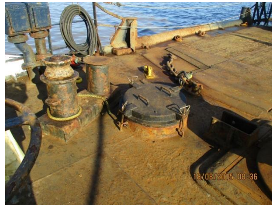
Main deck showing signs of aging but still acceptable
