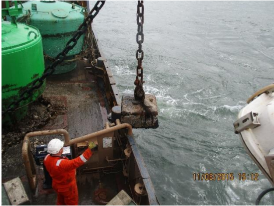
The sinker being lifted and checked
