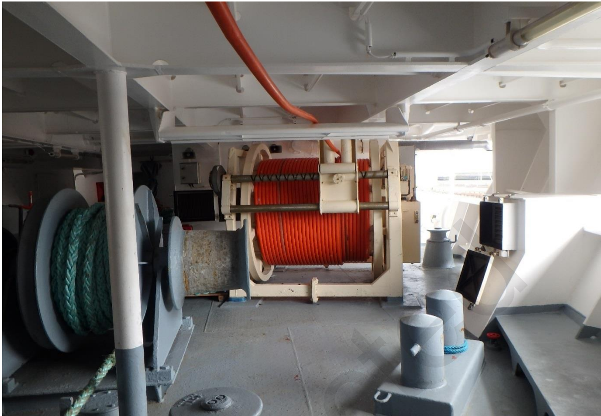
Photo 30 Fuel hose for supply to remote locations.
