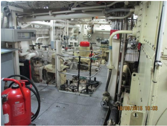
General Engine room photograph showing the condition
