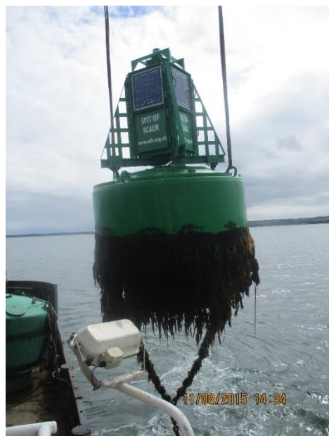
The Type 2 buoy lifted from Loch Ryan for cleaning and for the chain to be gauged.
