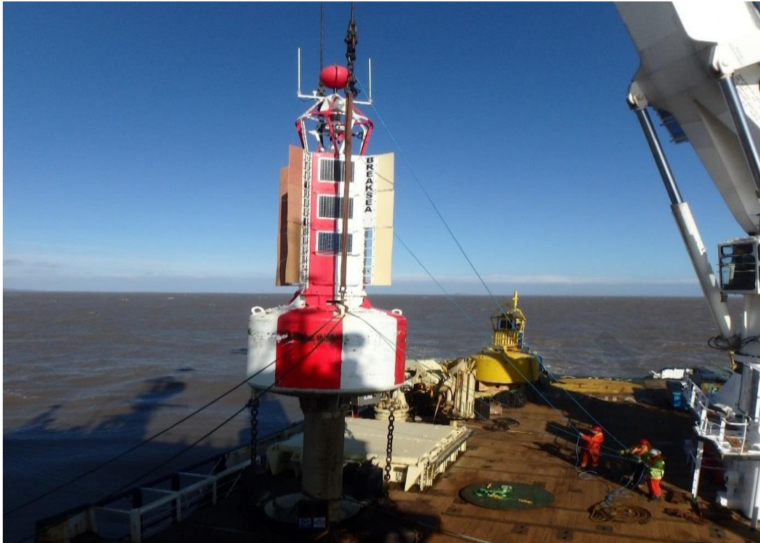
Photo 6 Starting to redeploy the Breaksea buoy after maintenance and cleaning. Once the buoy had been put back in the water, it was very noticeable that the buoy was moving about considerably and the crew on Galatea were very aware of the potential dangers of damage to the buoy which would not necessarily be the case if a TPV was chartered.
