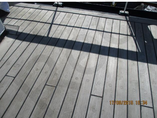
The accommodation decks are in very good condition
