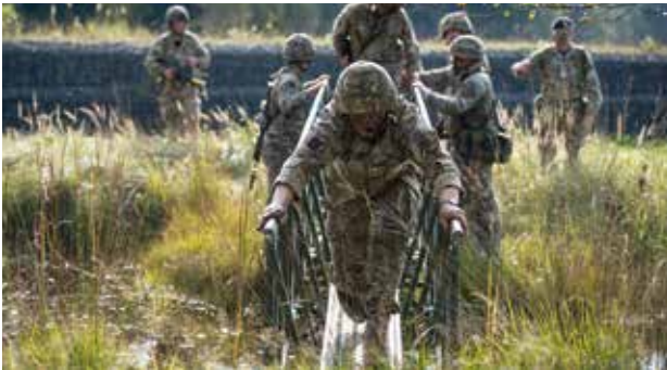
Reserve Engineers from 75 Engineer Regiment building bridges in Germany.
