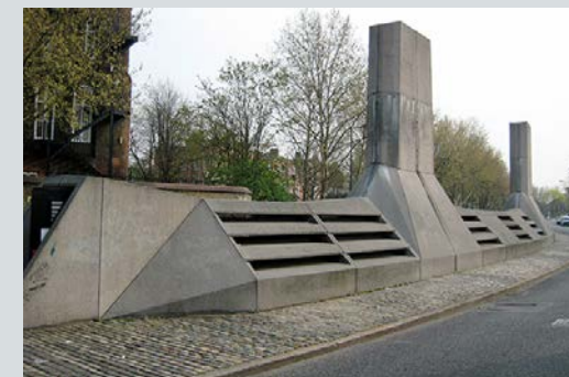
The "submarine" housing the CHP at Myatts Field North
