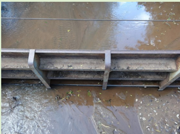
Siltation of the Tangadzi River contributed to the old head works in Muona falling into disuse.
