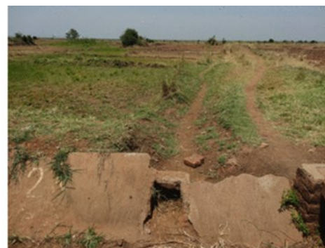
A section of Block E in Muona Irrigation Scheme showing a damaged secondary canal and a poorly maintained tertiary canal. Such poorly maintained canals are problematic when it comes to delivering water around the block once the farming starts.
