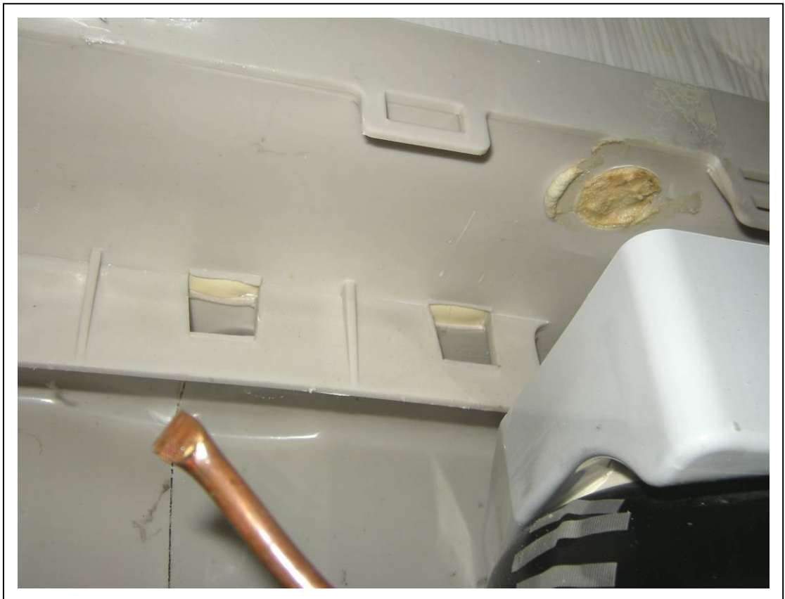
View of insulation foam visible at roof of compressor cavity
