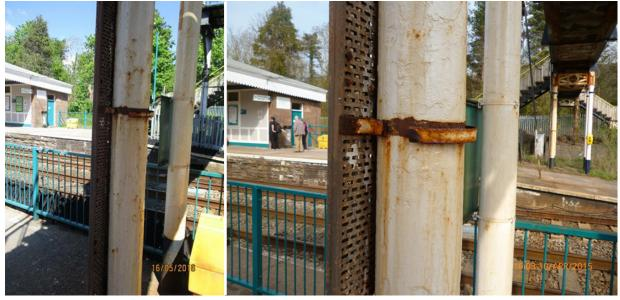
*Figure 21: Photographs of the cable tray bracket defects found during the last detailed inspection in May 2016 (images courtesy of Network Rail)*
