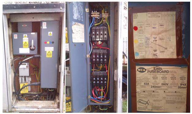
Figure 18: Photographs showing the main distribution board in the distribution cabinet (images courtesy of Arriva Trains Wales)
