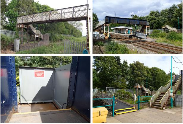
Figure 8: From top left clockwise: The footbridge lattice span, the footbridge after the lattice span had been removed, the temporary walkway to platform 2 over the disused lines and the footbridge corner section (top left image courtesy of Network Rail)
