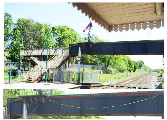
Figure 20: Photograph of the footbridge taken during the last detailed inspection in May 2016 with drooping electrical supply (red) and telecommunications (yellow) cables (image courtesy of Network Rail)
