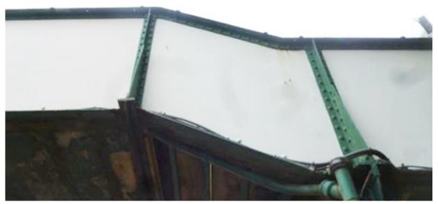
Figure 24: Cables routed on the outside of the footbridge at Helsby station (image courtesy of Network Rail)
