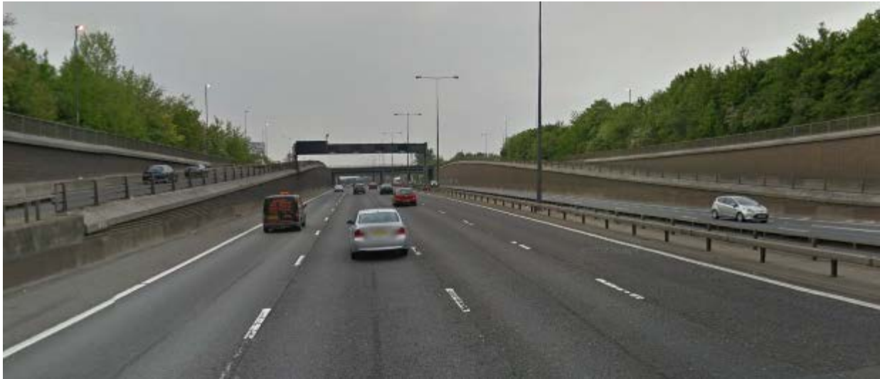
Image 1 – A282 northbound approaching Junction 1b showing examples of retaining walls, bridges and constrained carriageway
