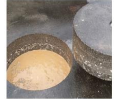
↑ Figure L: Removal of the core (Source: Tracto Technik)
