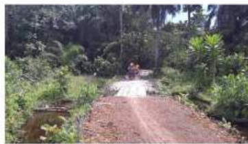
MCTs riding over newly constructed trail
