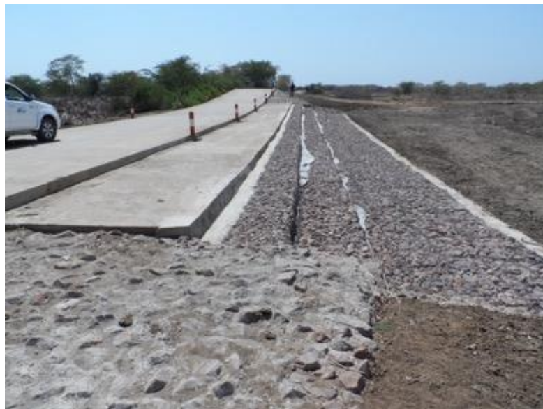
Figure 3: Concrete ford with stepped gabion protection baskets
