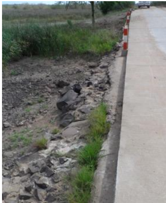
Figure 20: Erosion of stream-bed to left of ford at km 34.8
