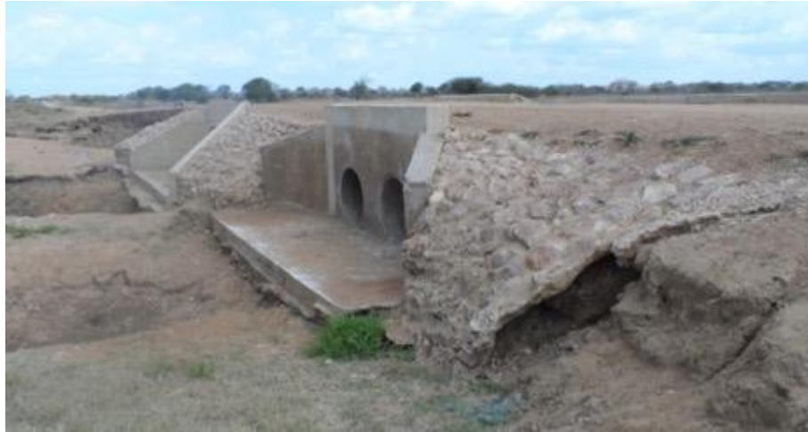
Figure 28: Damaged protection works at km 10.6
