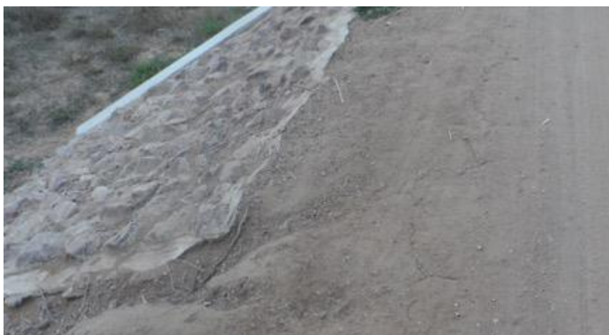
Figure 30: Cracking of material in embankment at km 10.6
