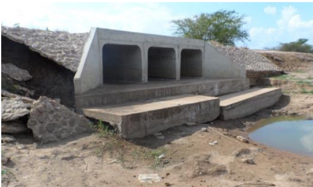
Figure 18: Damage to culvert at km 33.4
