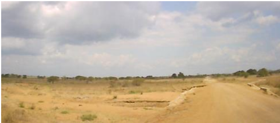
Figure 29: Approach to the two culverts at km 10.6 from north
