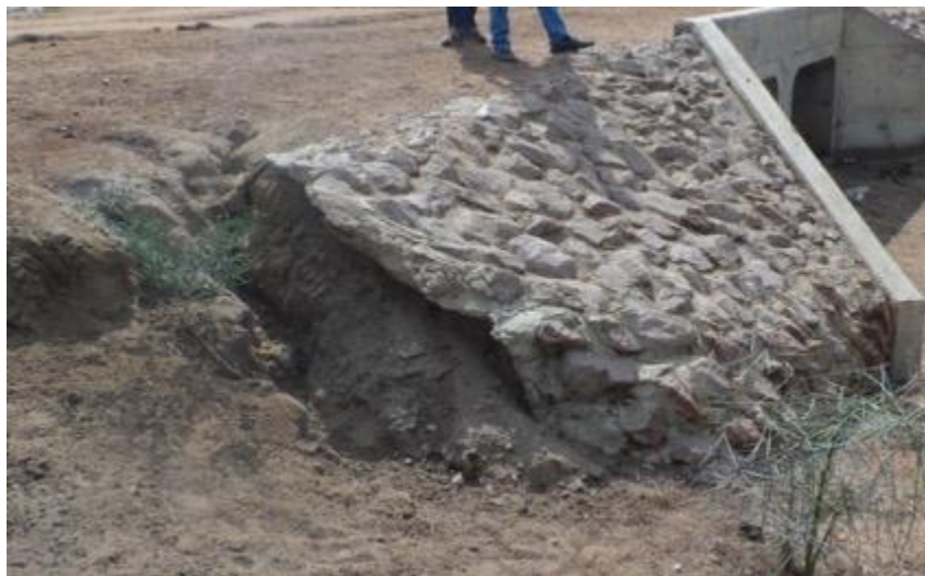
Figure 32: Erosion damage at edge of stone pitching
