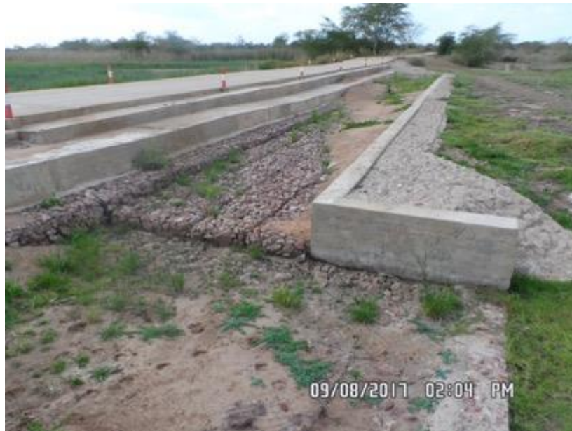
Figure 22: Accumulation of sediment in water-traps of ford at km 34.9
