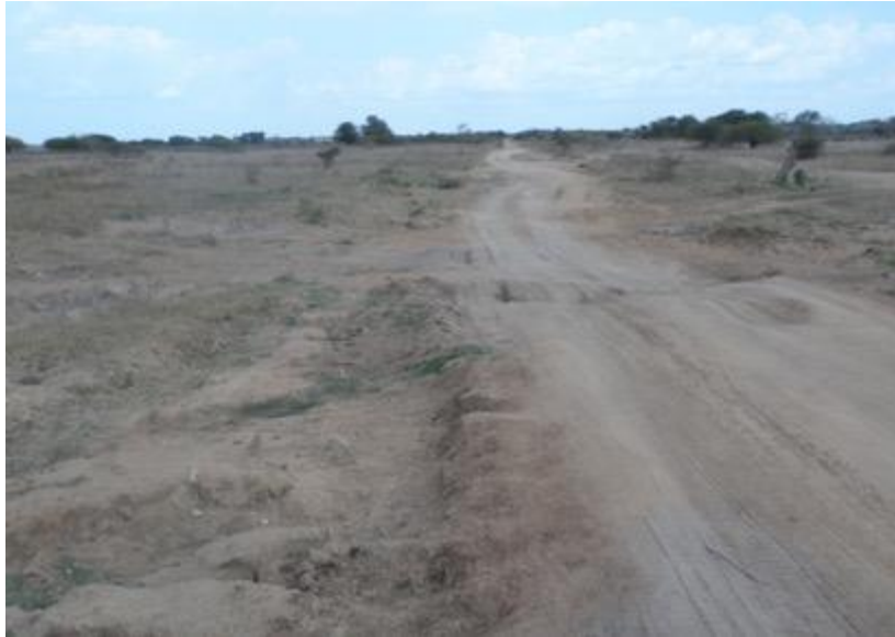
Figure 33: Area of crossing water that misses the culverts – the water moves from the right to the left and then almost parallel to the road to re-join the stream below the two culverts, causing a lot of the erosion.
