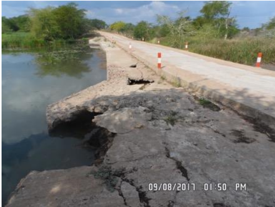
Figure 19: Damage to ford protection works at km 34.8
