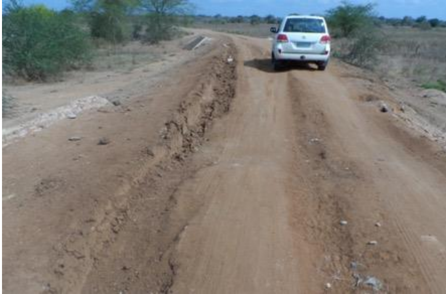
Figure 15: Deformation of road between the two culverts at km 24.9
