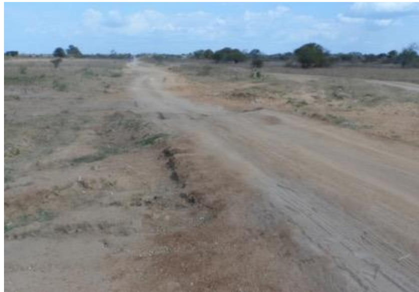
Figure 10: Southern approach to culvert
