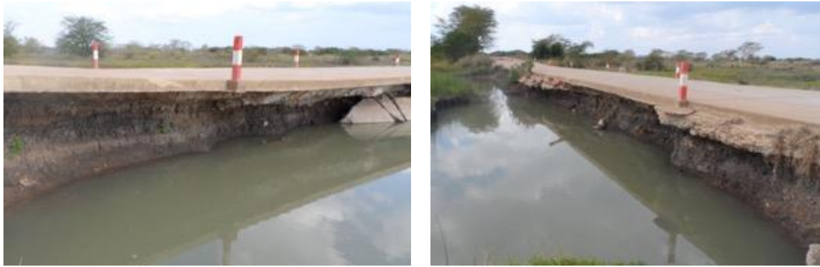
Figure 21: Undercutting of ford at km 35.9
