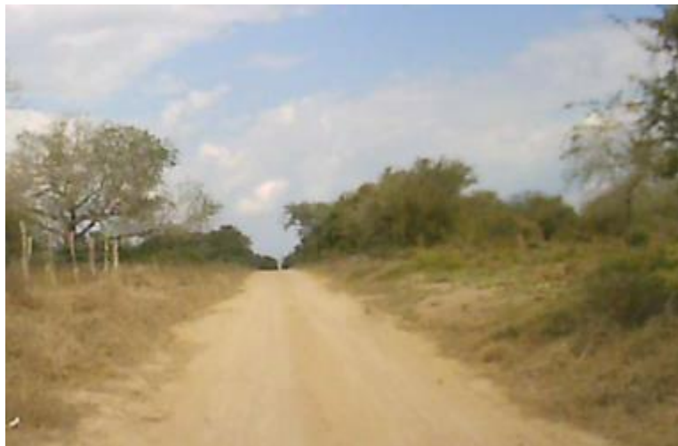
Figure 14: Narrow road in a channel with no drainage (km 23.8)
