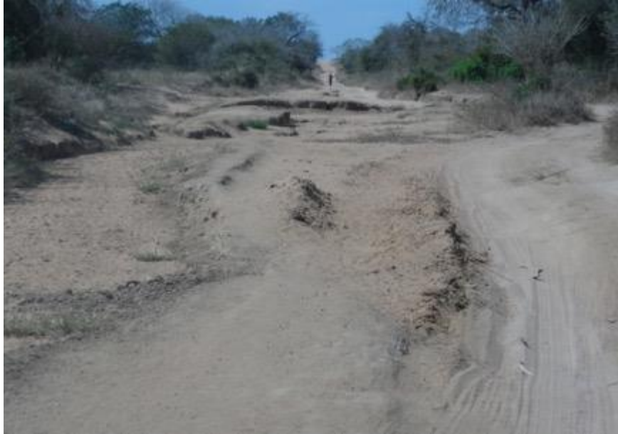
Figure 11: Erosion damage to road at km 15.8
