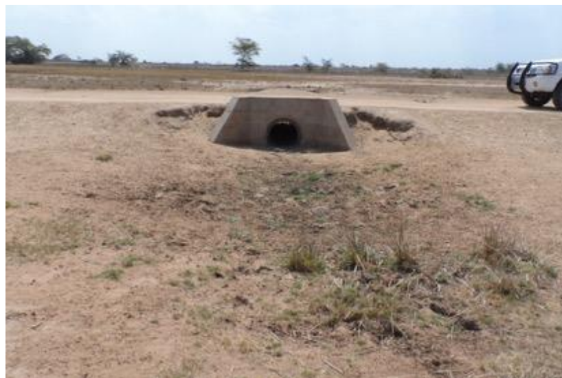
Figure 5: Culvert in flat terrain
