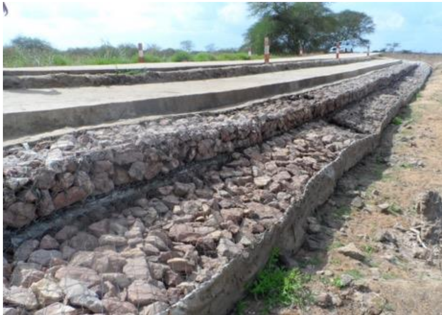
Figure 12: Deformation of damaged gabions
