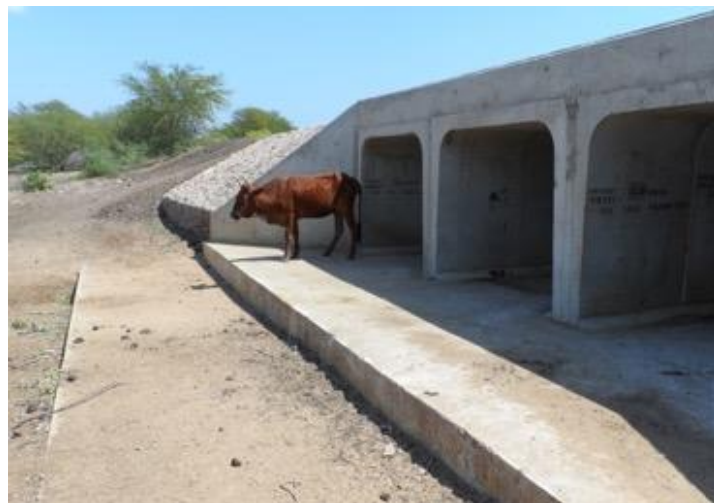
Figure 7: Culvert constructed under emergency repair programme in 2014)
