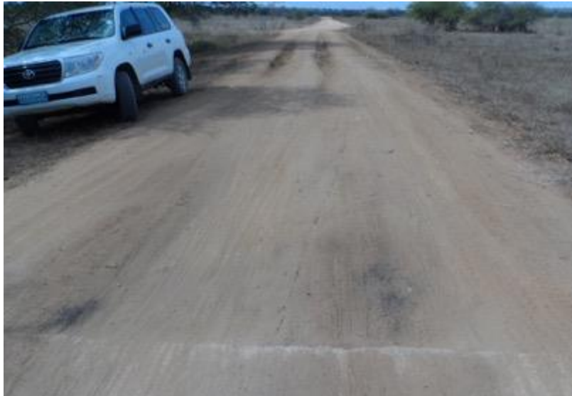
Figure 13: Erosion, subsidence and deformation of northern approach to ford
