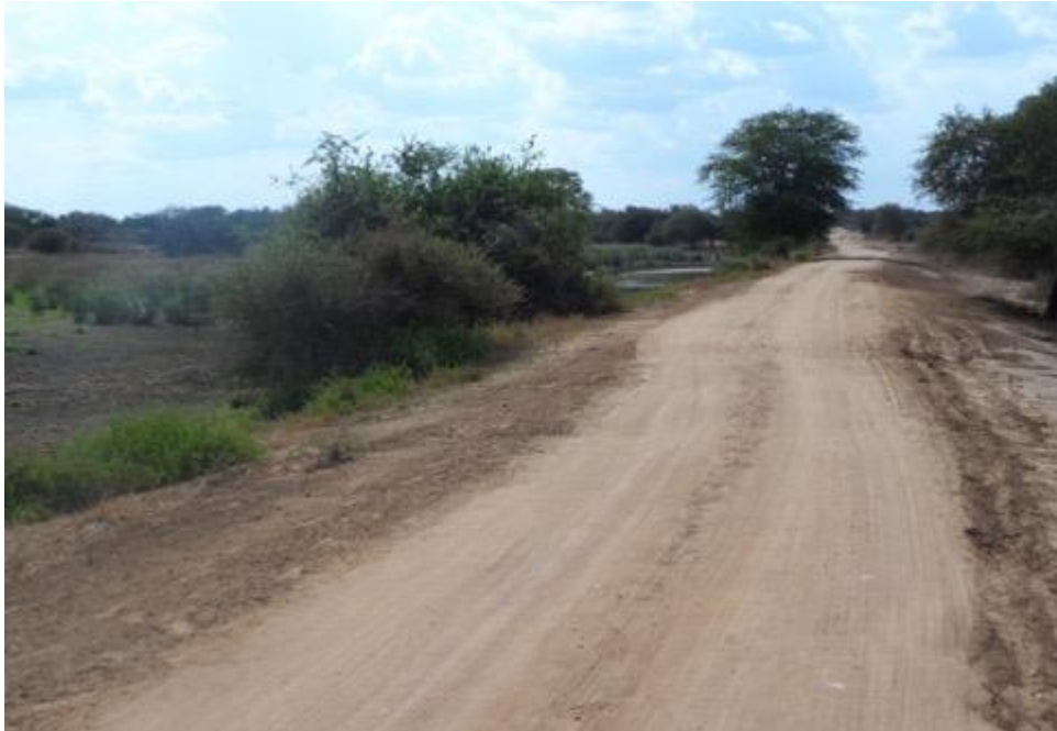
Figure 16: Dam next to road which overflows damaging road – channel on left side requires modification
