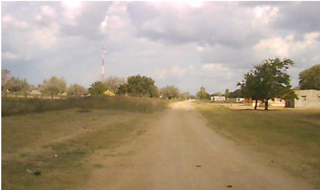
Figure 24: Proposed demonstration section for 200 m up to culvert just past start of sunny area
