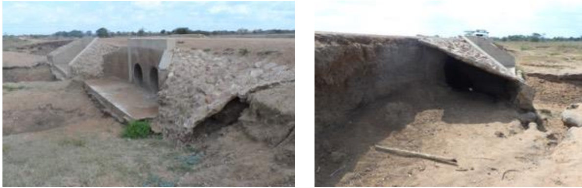
Figure 9: Damage to structure and erosion protection measures at km 10.6
