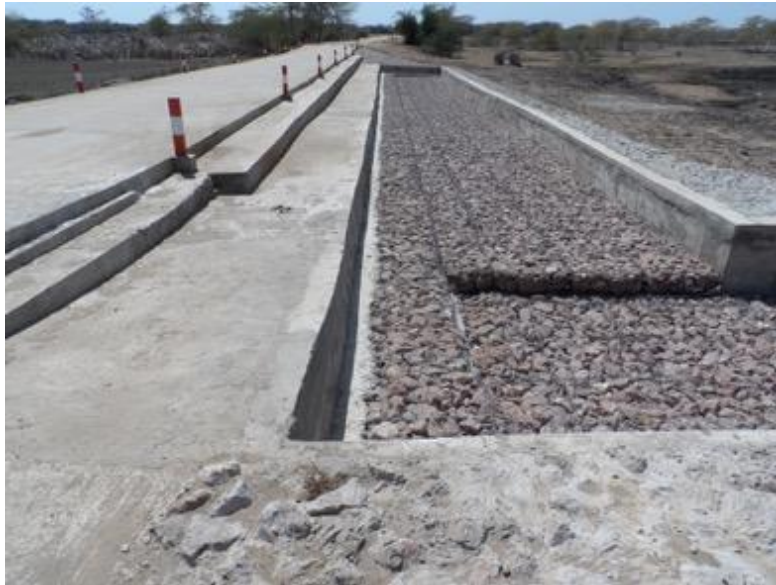
Figure 4: Concrete ford with gabion lined stilling pond to minimise water velocities and erosion
