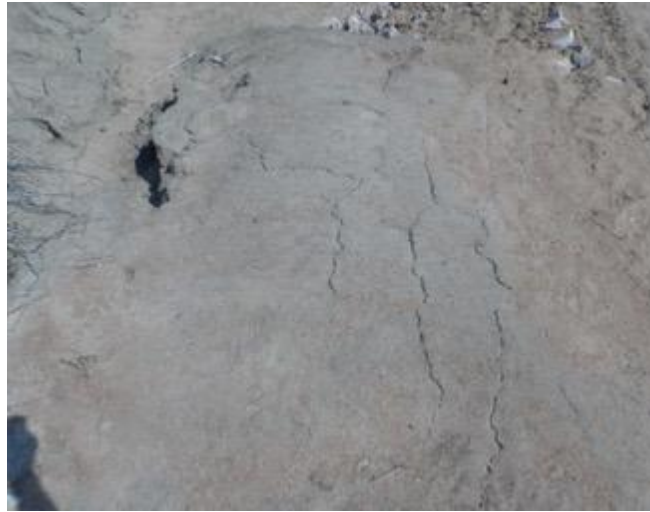
Figure 17: Cracking of exposed in situ material in shoulder area of road with erosion at left top
