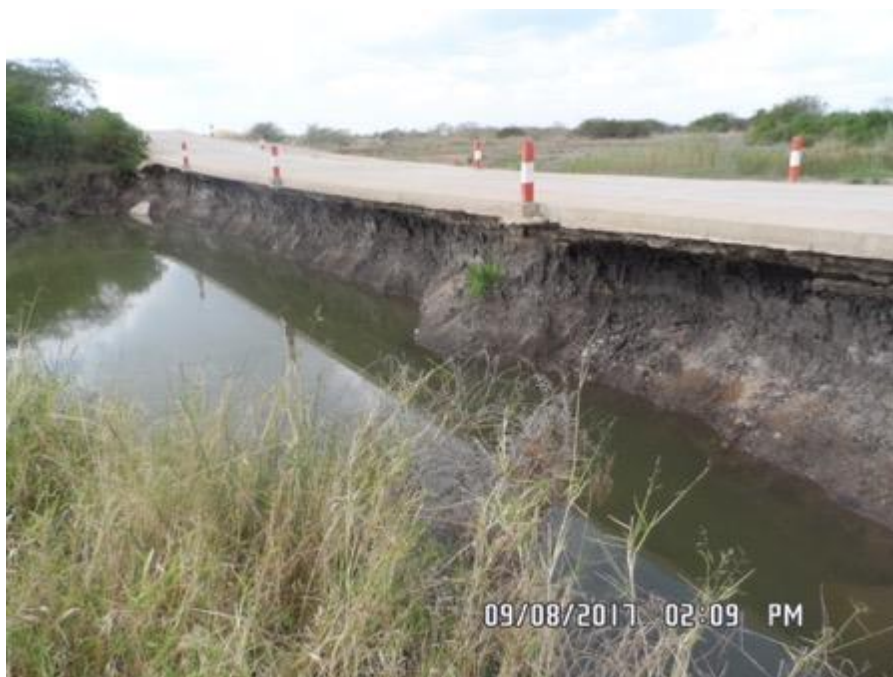
Figure 23: Undercutting of ford at about km 36
