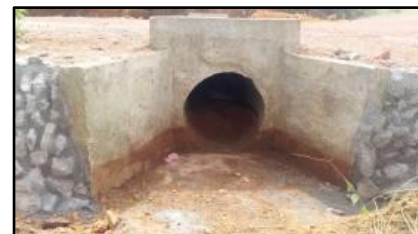
Stone Pitching of embankment slope
