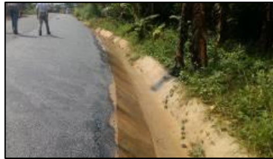
Concrete lined trapezoidal drain
