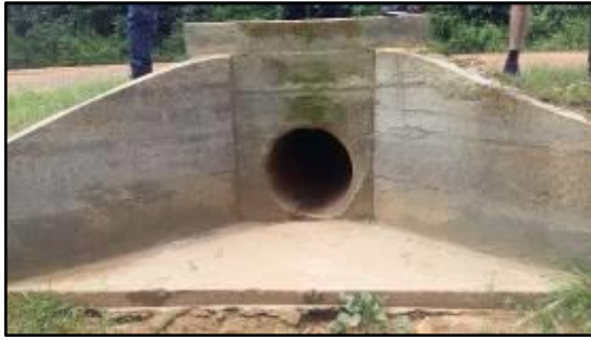
Well-constructed cross culvert with apron
