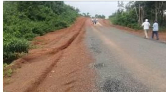
Mitre drain/turn-out at steep slope
