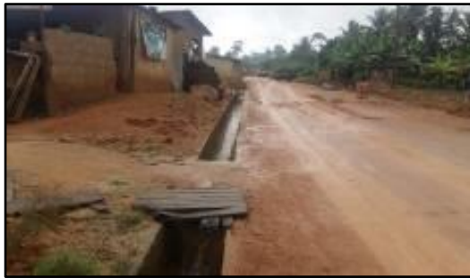
Concrete lined u-drain
