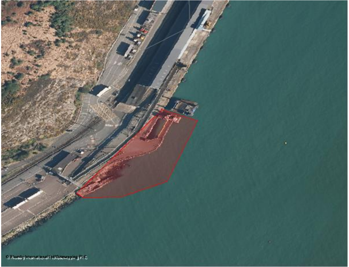
Figure 1: Fishguard Linkspan Replacement
