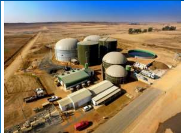
Bio2Watt Bronkhorstspuit biogas plant, South Africa
