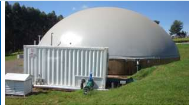
James Finlay Kenya biogas plant, Kericho
