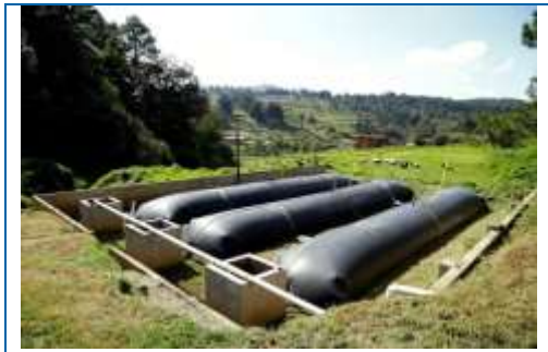
Sistema Biobolsa installation in Mexico
