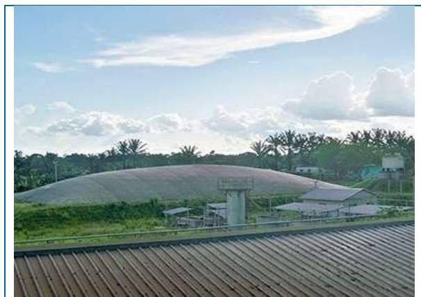
Siat palm oil waste biogas plant, Makouké, Gabon
