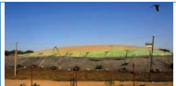
Fasobiogaz biogas plant, Ougadougou
