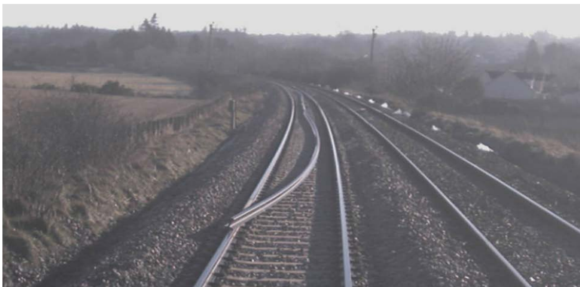
CCTV image showing the rail on the track shortly before the train struck it (image courtesy Virgin Trains East Coast)
