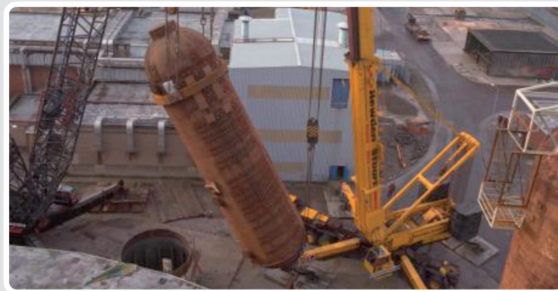
Removal of Berkeley boilers (Magnox)
