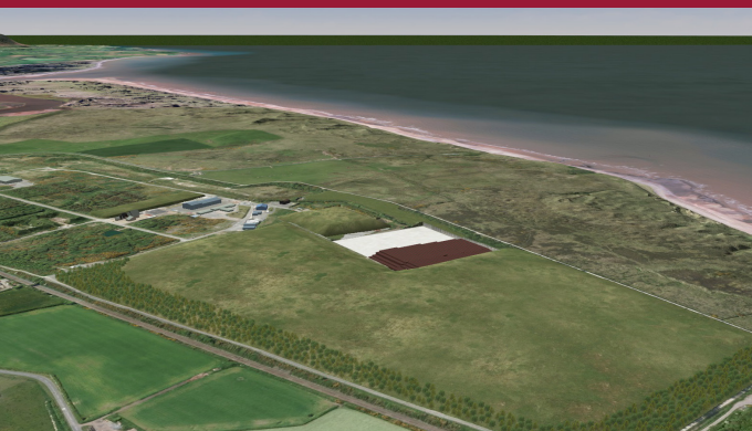
Phase 3: 2023 — 2030: Capping of Vault 9 and adjacent trenches, construct Vault 11
