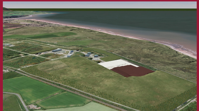
Phase 2: 2019 — 2023: Capping of Vault 8 and adjacent trenches construct Vaults 9A+10
