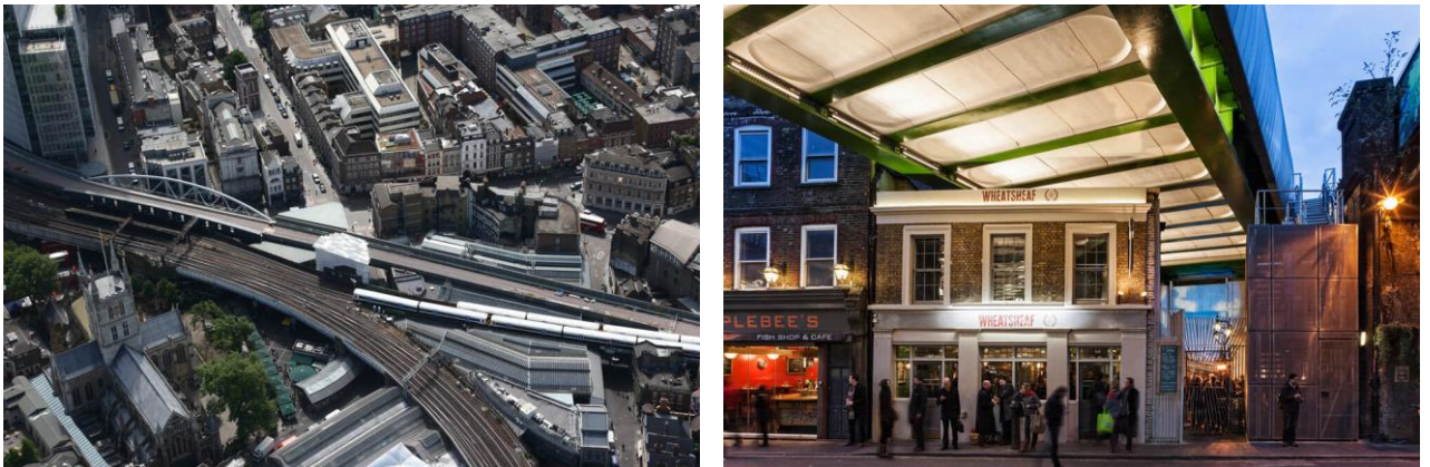
Figure 6 Borough Viaduct (aerial view and ground view)
