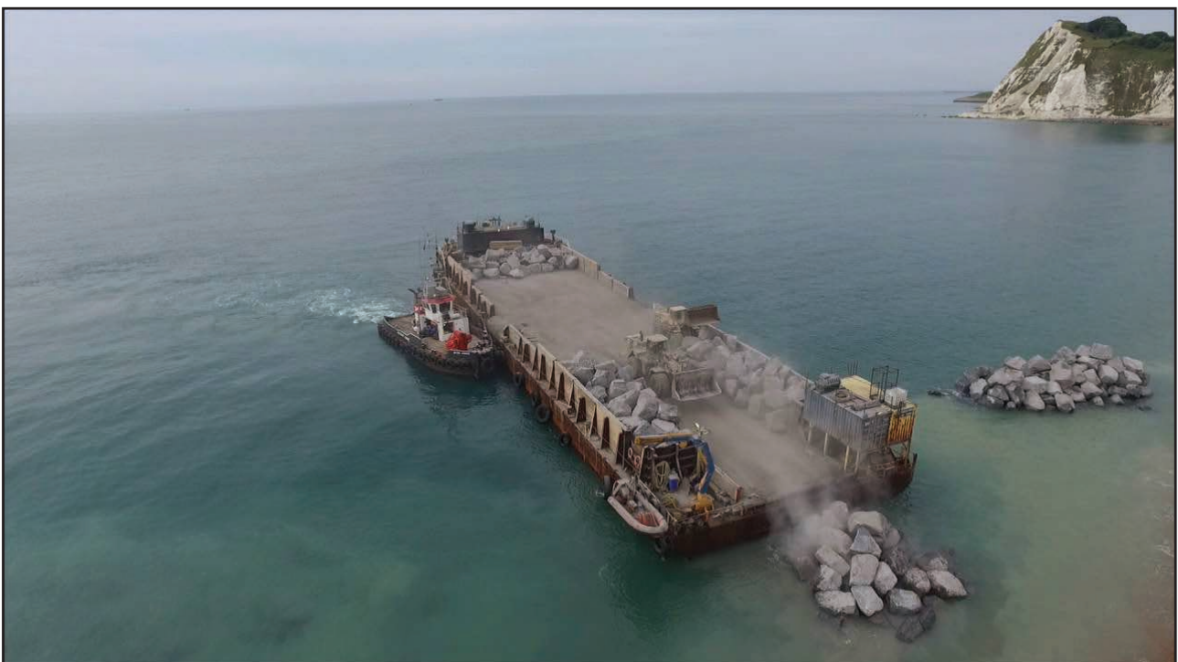
Figure 7b: Charlie Rock discharging rock armour
