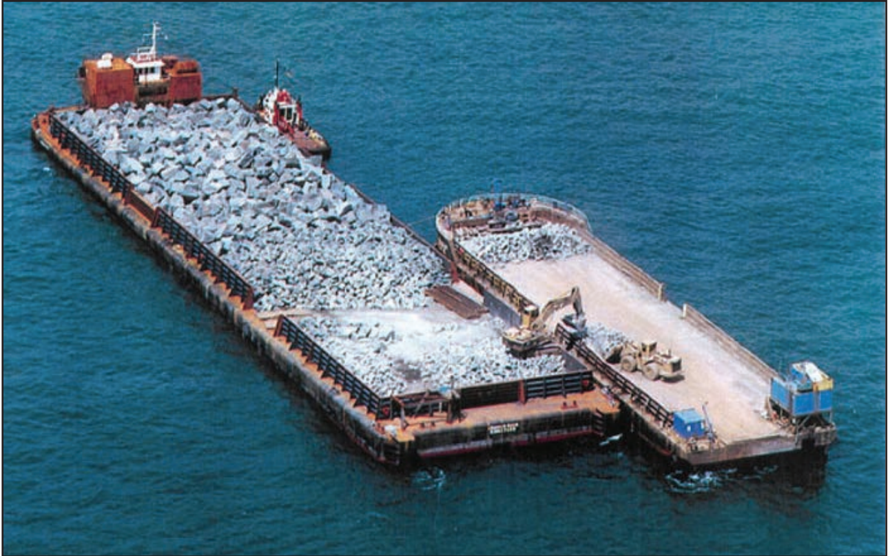
Figure 7a: Stema Barge II transferring rock to Charlie Rock
