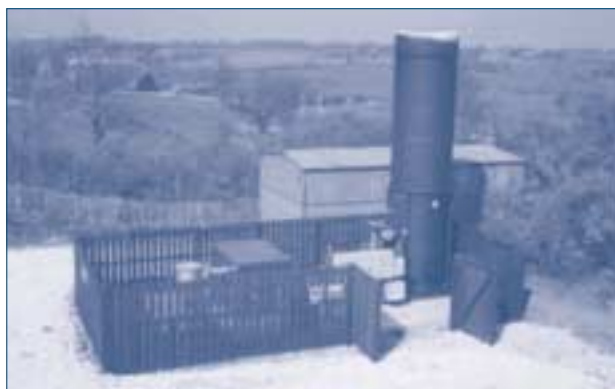
Figure 4.3 | Enclosed flare station
