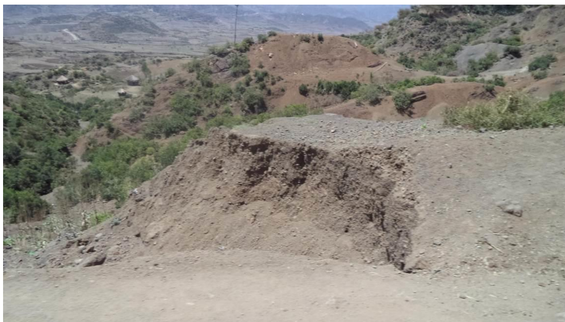
Figure 16: “This stretch of the road (connecting Kebele 28 to Kobo town) gets eroded every season. Vehicles can easily fall down the hillside.”- Image by Photo Voice group from Kebele 28 (women group) on 7-3-2017.
