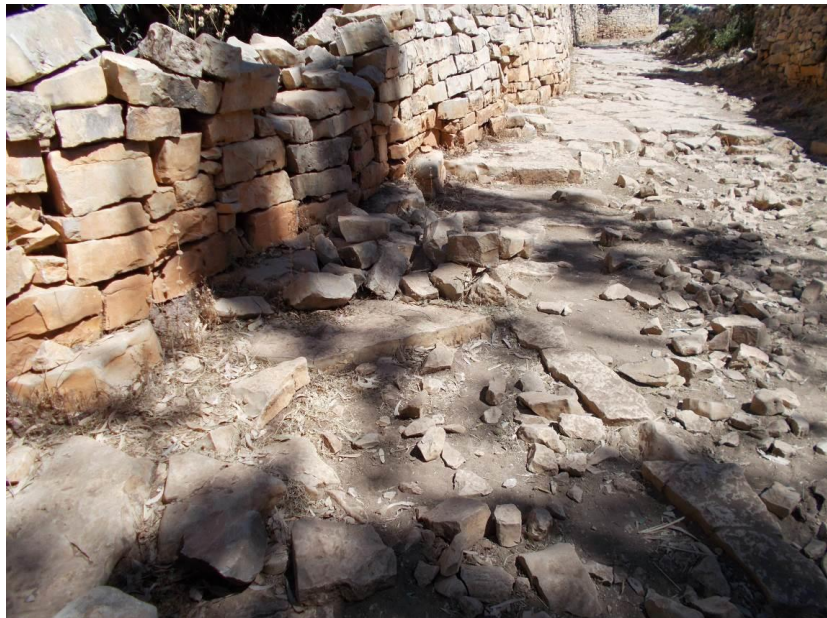
Figure 17: A rocky 'First-Mile' stretch in Aynalem village
