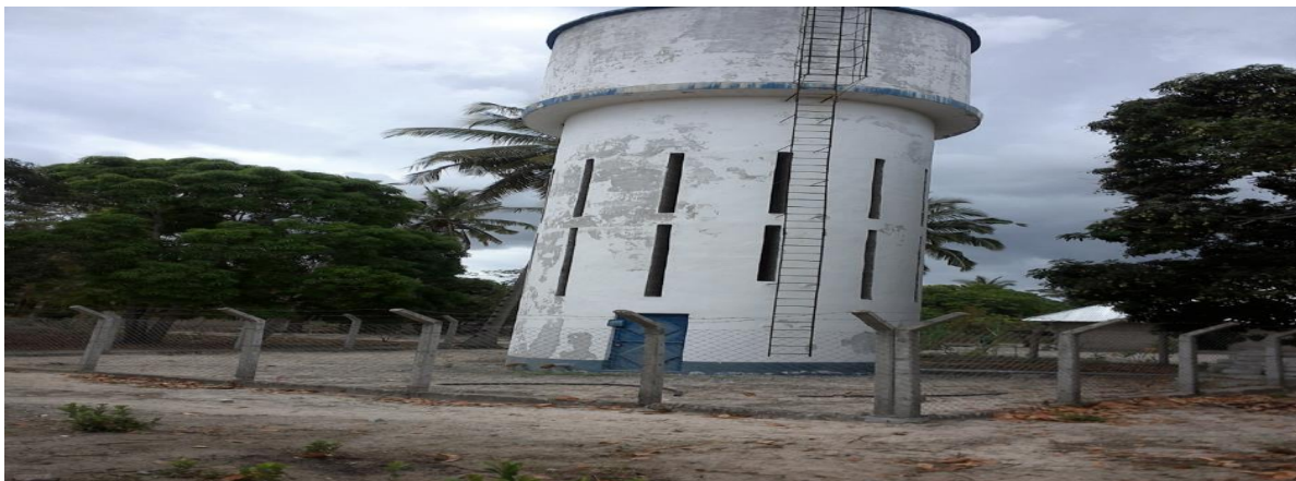
Case 16: Water Supply Infrastructure (Tank) built besides the Makazi-Mapya Ngeta Road. The water tank accommodates 100,000 litres of water and serves 7 villages.
