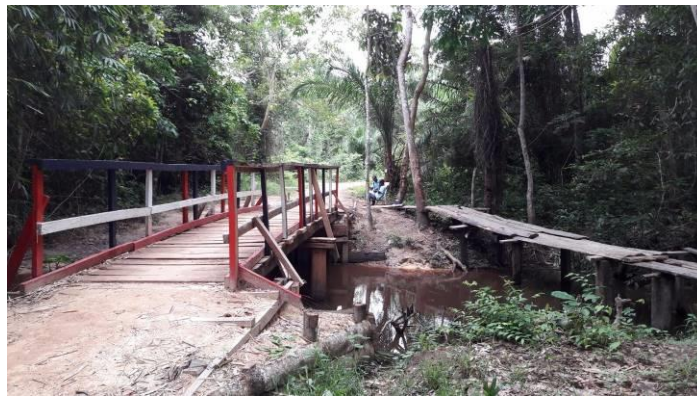
Figure 4 - Newly constructed bridge at the Global Communities built motorcycle navigable track next to the old footbridge, near Gogein, Nimba County, Liberia.
