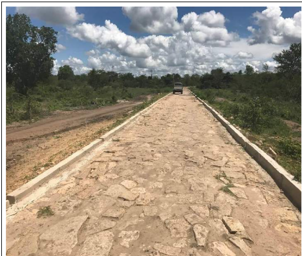
Deformations and loss of stones
