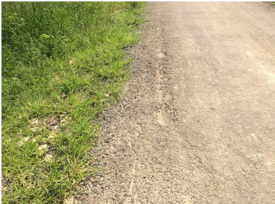
Stone loss and exposed geogrid, drains covered by shrub, tall grass
