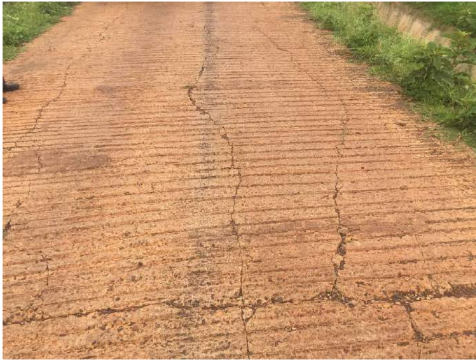
Dominance of longitudinal cracks, vegetation growth on the shoulders
