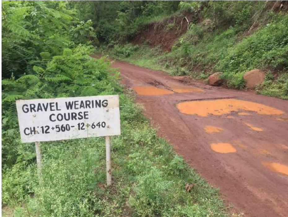
Water ponding, potholing.
