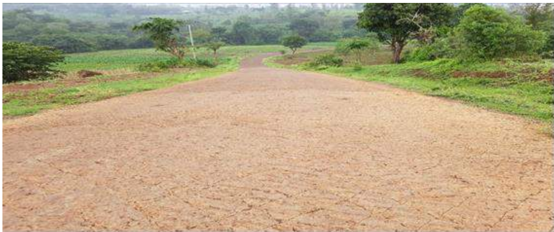
Geo-cell surfacing performing very well.
