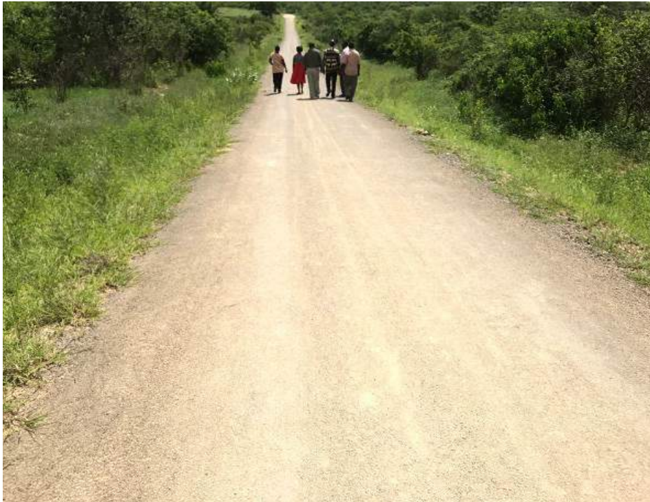
Good performing section, drains covered by shrub, tall grass
