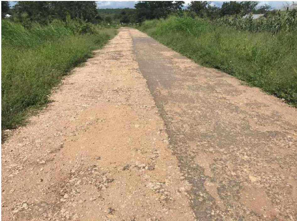
Performance of cement slurry seal (RHS) relatively better than lime slurry seal (LHS), Shoulder failure, drains covered by shrub, tall grass
