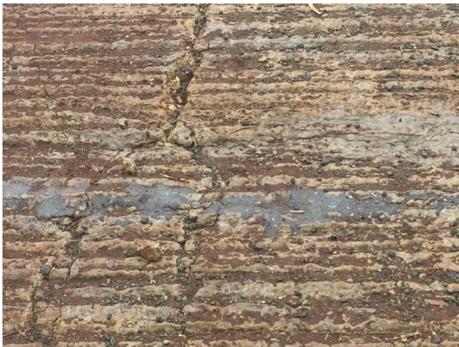
Close-up of longitudinal cracks
