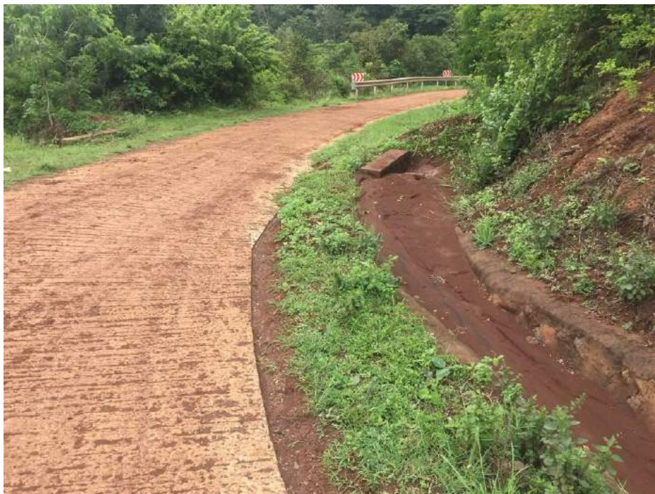
Surfacing performing very well, but severe sedimentation build-up
