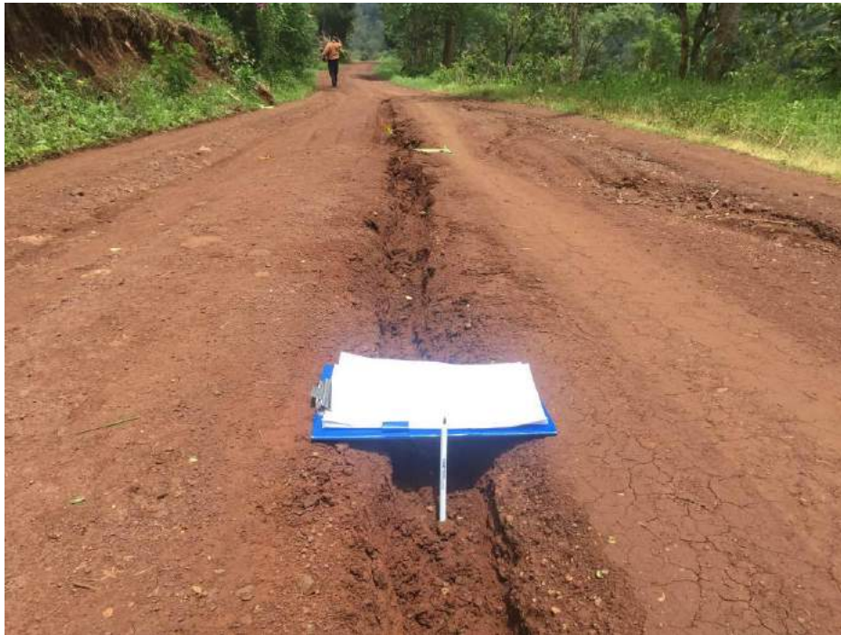
Severe erosion tracks
