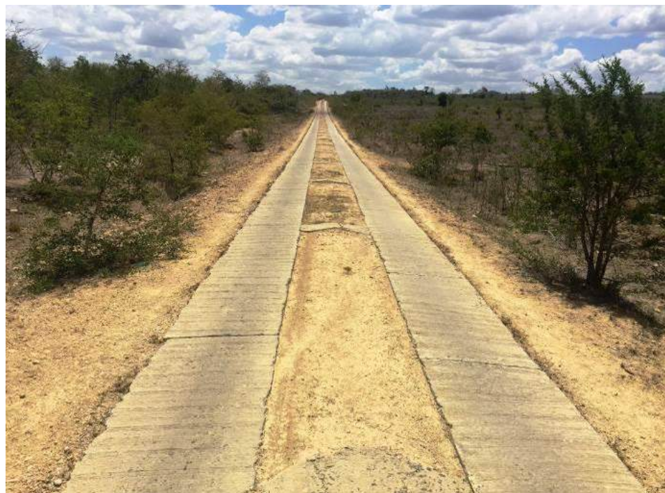
Concrete strip, gravel shoulders severely eroded
