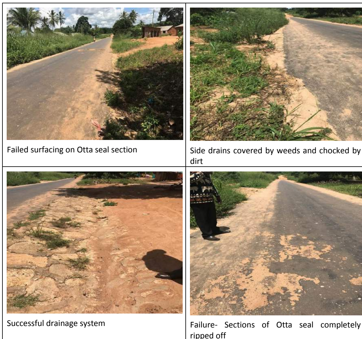
Figure 5: Observations on Otta-seal sections
