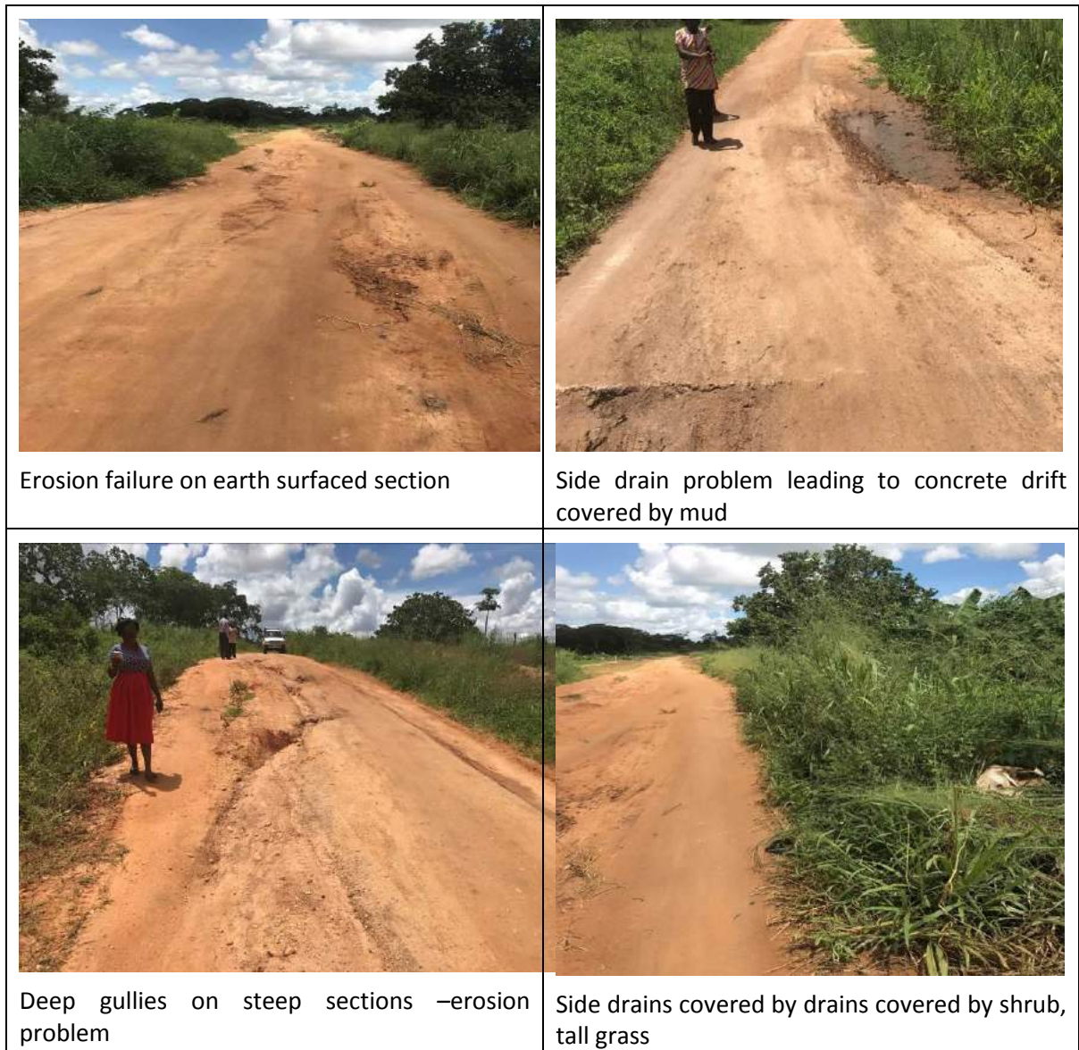
Figure 6: Earth surfacing sections
