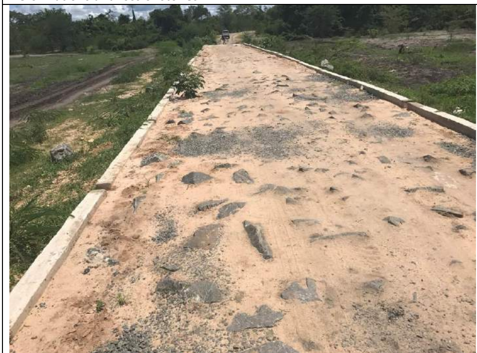
Severe stone loss
