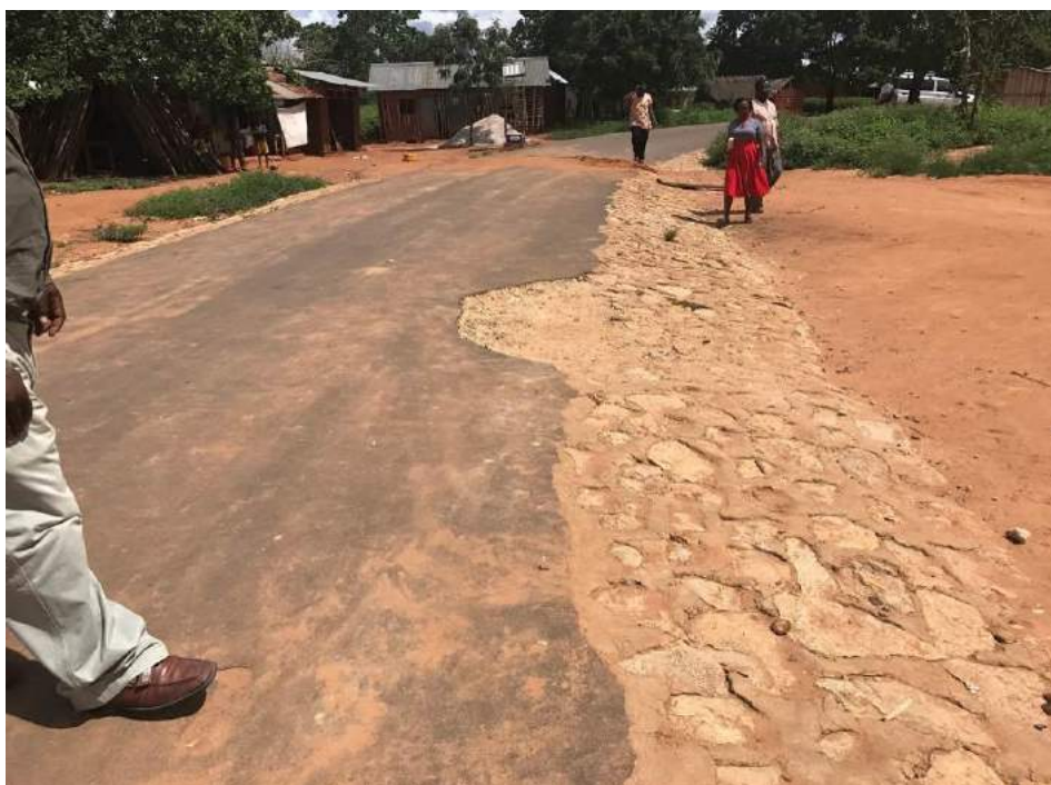
Shoulder failure
