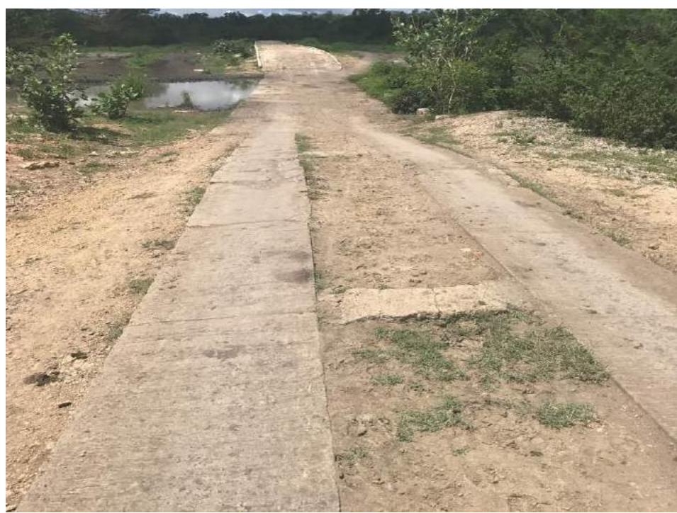
Failed concrete strips (cracking, erosion, gravel loss between strips, etc.)
