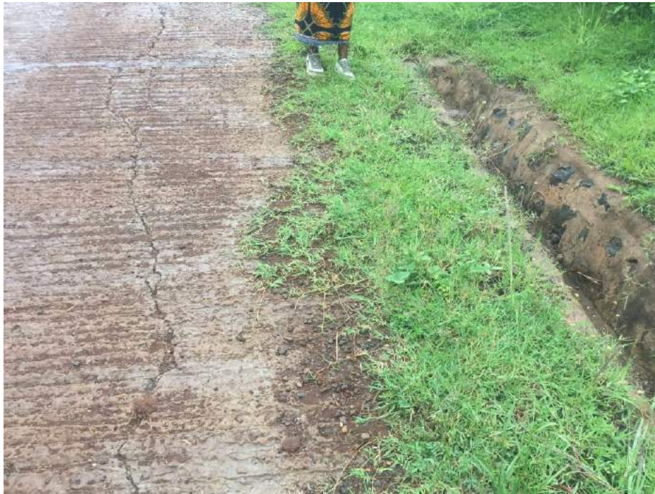
Longitudinal cracking, vegetation growth on shoulder, clean drain
