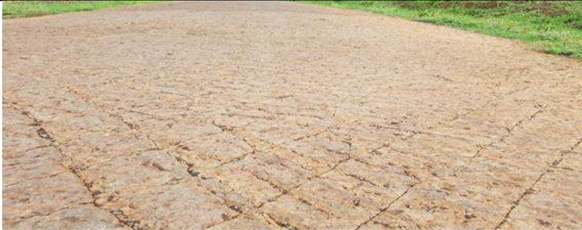
Showing compactness of Geo-cell surfacing
