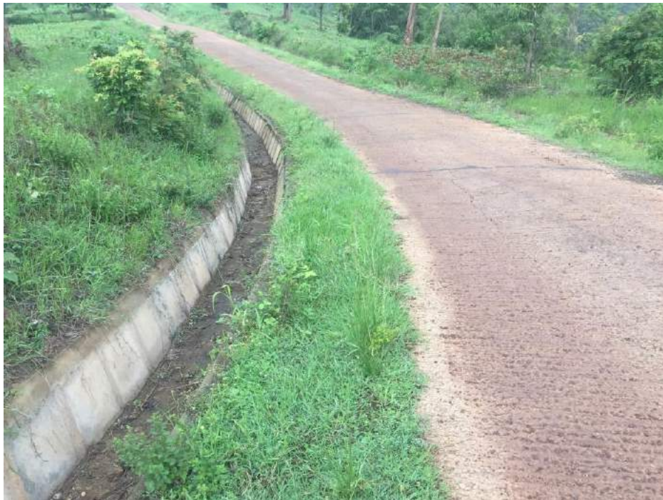
Sedimentation build up, vegetation growth on shoulders
