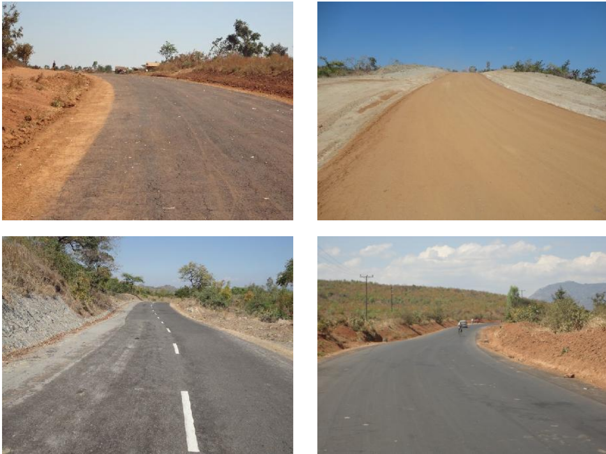
Figure 1: Examples of completed and ongoing works on the three project roads
