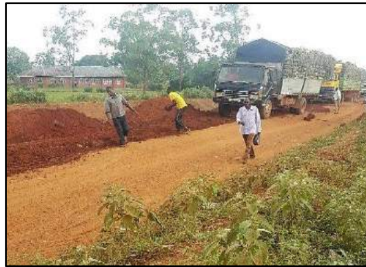
Figure 9: Murrum dumped on the road in Namwendwa
