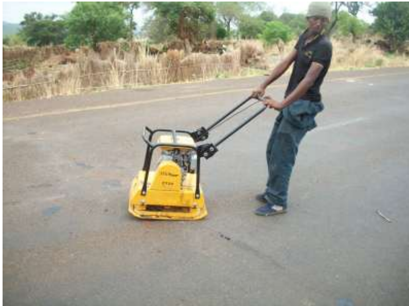
Figure 2-3: Reinstating works after DCP test
