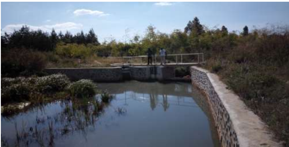
Figure 22: Irrigation Dam Control Point at Mtula area
