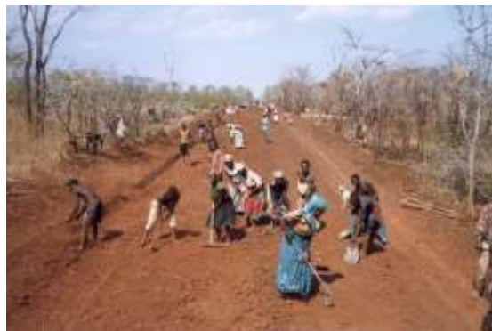
Figure 5: Labour Based Road Construction
