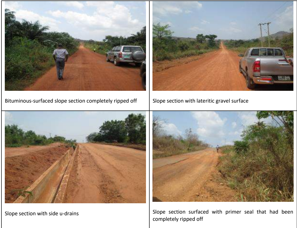
Figure 13: Some terrain features of Akosombo– Jakiti road
