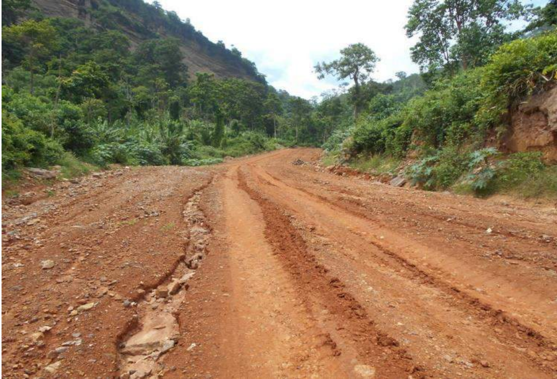
Figure 23: Early erosion signs of road surface due to steep slopes on gravel surface
