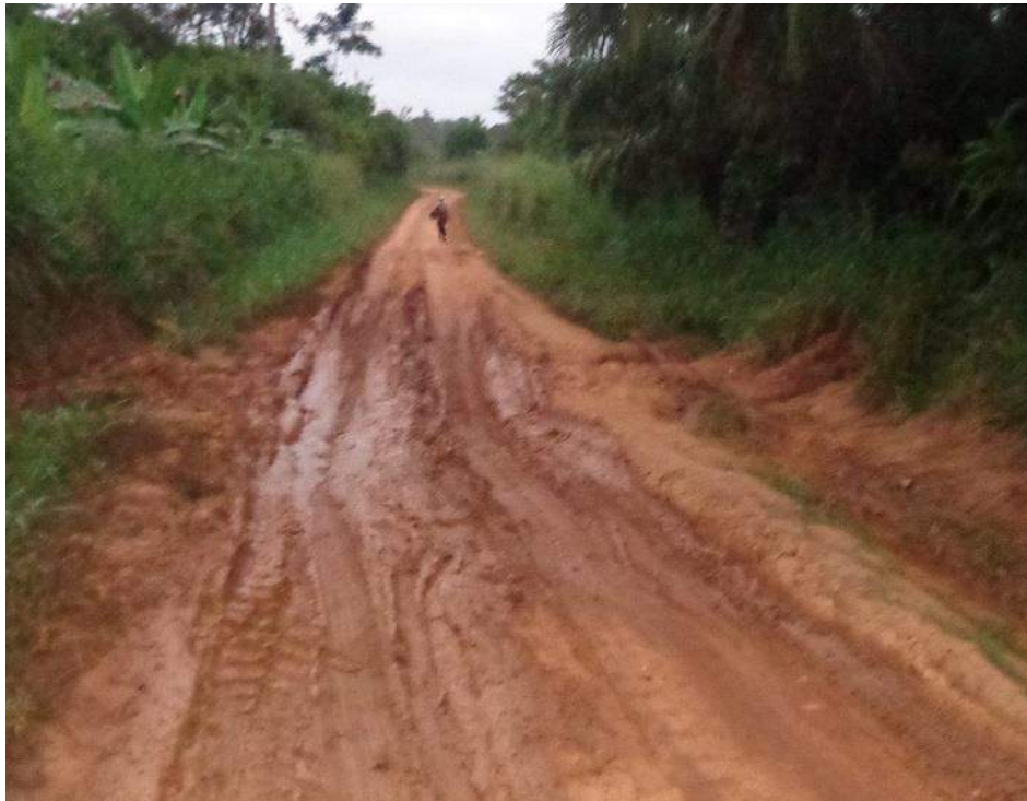
Figure 1: Road section requires proper drainage /surfacing intervention
