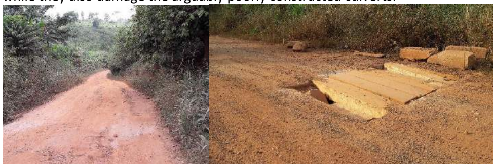
Figure 5 (left) – Deteriorated road section of one of the feeder roads
