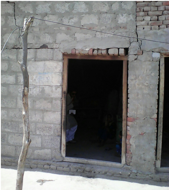
Figure 08: Example of low strength wall
