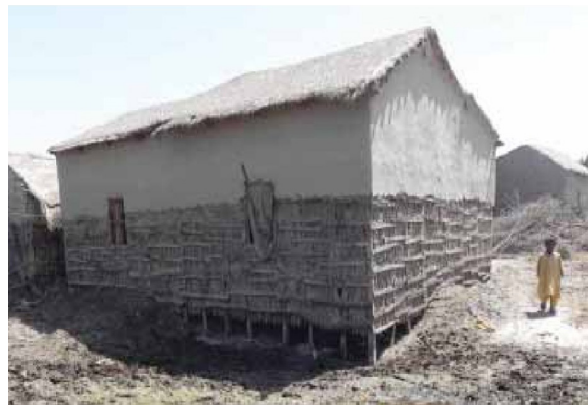
Figure 15: Example of flood damage to loh kat shelter
