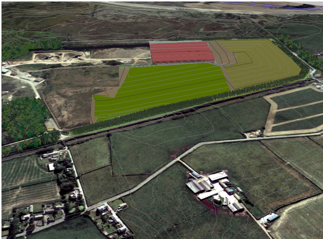
Figure 3.2 Vault 8 final capped
