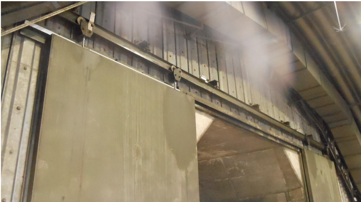
Photo 1 Showing efflux door, runway beam and supporting brackets
