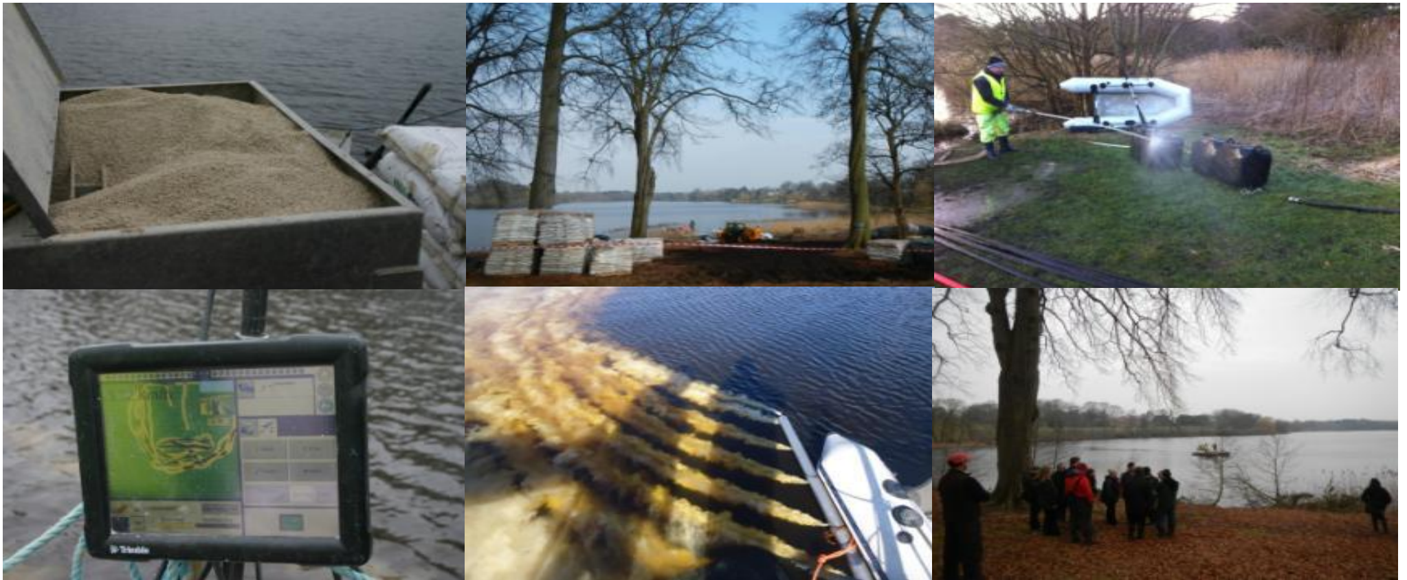
Figure 2.2 Photographs documenting the Phoslock® applications at Hatchmere and Mere Mere. From top left: Phoslock® in the hopper prior to slurry application; product being loaded from shore onto the pontoon at Mere Mere; cleaning of equipment following application as part of the biosecurity measures. From bottom left: product application track; plume of product during application; site visit by project board and stakeholders at Mere Mere during application
