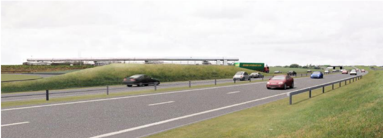
Figure A.14 – Recreation of photomontage from Figure 2.11e from ES. Representative View (Turnpike Roundabout) taken during autumn 2010 (After scheme opening)
