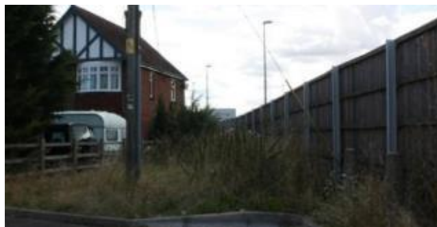
Figure 5.5 – 1.9m high environmental barrier at properties near Lady Lane Junction.
