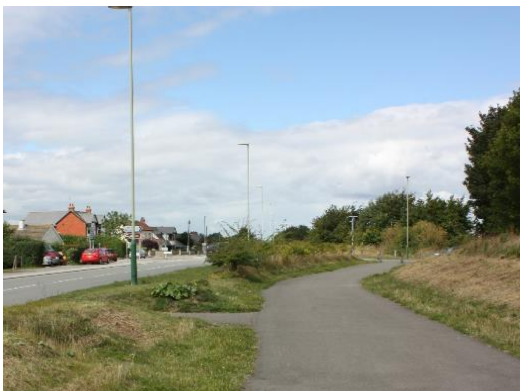
Figure 3.4 Footpath and Lighting on the former A419
