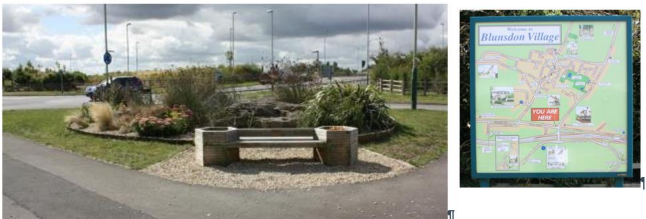
Figure 5.18 – Former A419 has been de-trunked and adopted by the Swindon Borough Council
