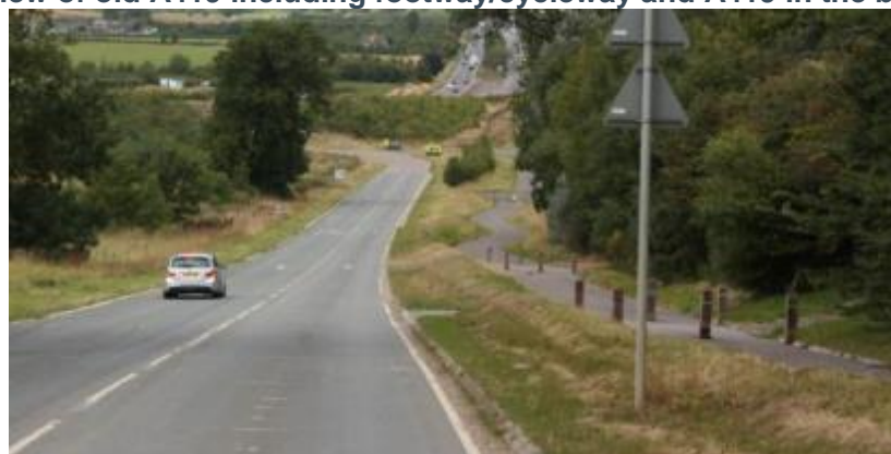
Figure 5.31 – FYA view of old A419 including footway/cycleway and A419 in the background
