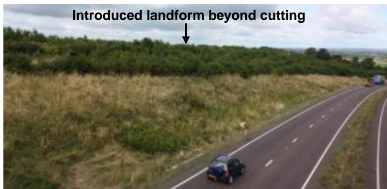
Figure 5.8 – View taken from Widhill Lane overbridge looking towards Upper Widhill Farm
