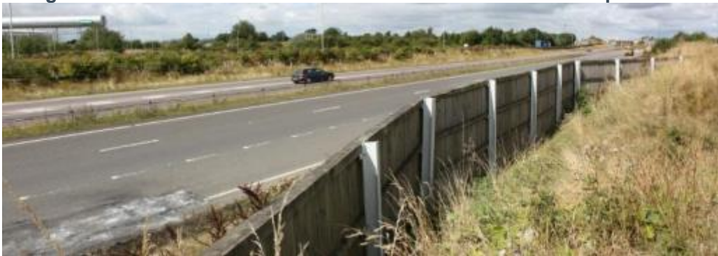
Figure 5.4 – Environmental barrier between the A419 and Turnpike Road
