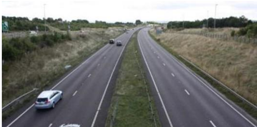
Figure 5.7 – View looking north from Lady Lane junction
