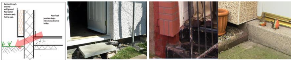
Figure 2-8 Thermal breaks introduced to ground floor/wall junctions where the EWI is stopped around 150mm above ground level. The examples show a 1970 terrace, a pre-1919 terrace and a 1950s semi
