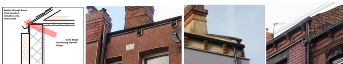
Figure 2-1 Thermal breaks introduced to top floor wall/ceiling junctions: pre-1919 terraces and back-to-backs
