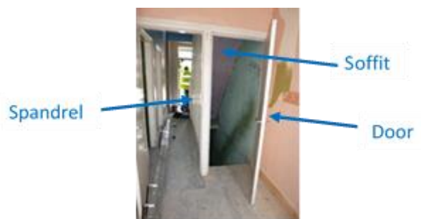
Figure 2-11 Interfaces between the unheated basement and heated ground floor which need to be insulated
