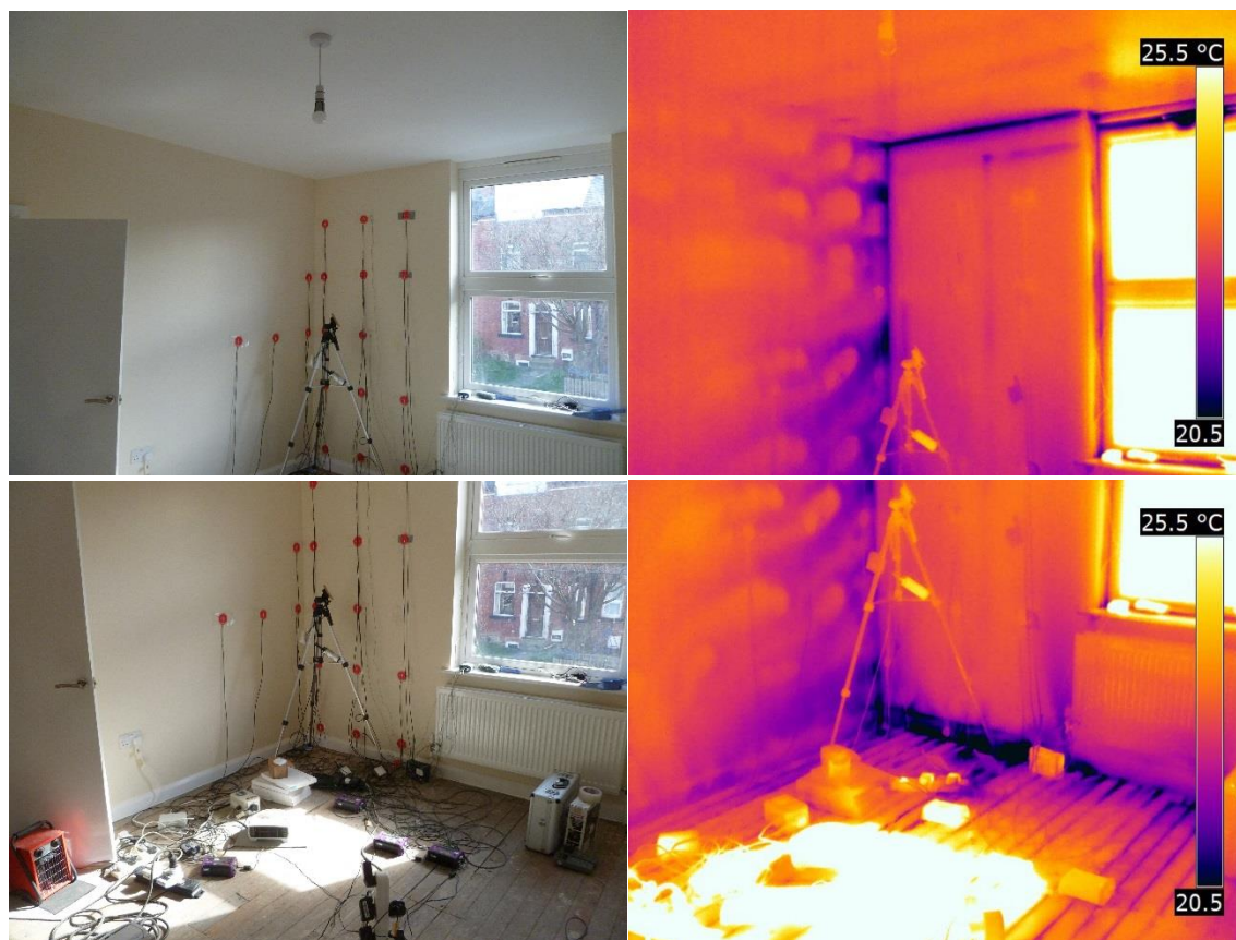
Figure 3-7 Dwelling C-02 under depressurisation following refurbishment.
