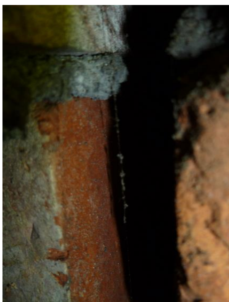
Figure 5-3 Cavity in Solid Brickwork External Wall
