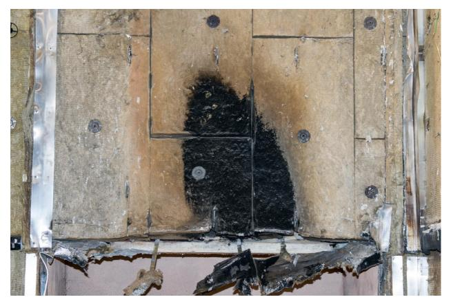
Figure 23. Close up of melted window pod and collapsed horizontal cavity barrier directly above the combustion chamber.
