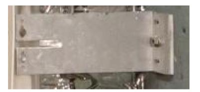
Figure 6. Example of aluminium rail fixed to 'L' bracket through movement holes.
