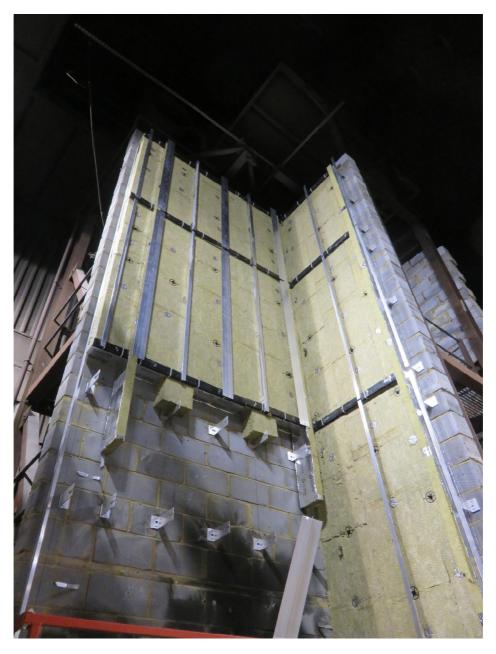
Figure 5. Partial installation of cavity barriers, stone wool insulation and railing substructure.
