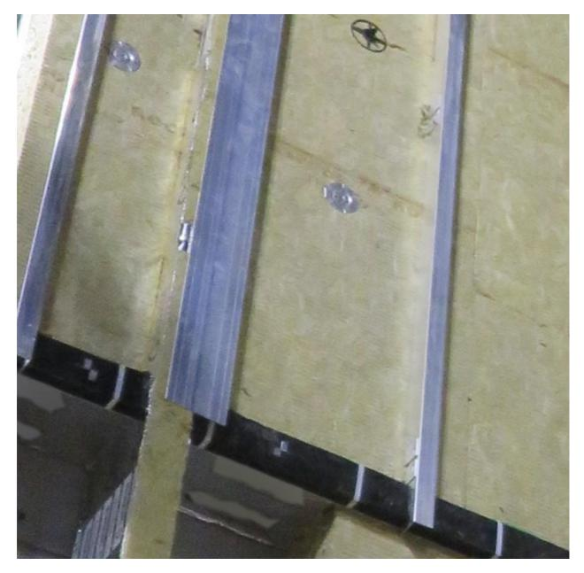
Figure 4. Horizontal intumescent cavity barrier fixed through the entire depth on face turned steel brackets, at the intersection with a vertical cavity barrier.
