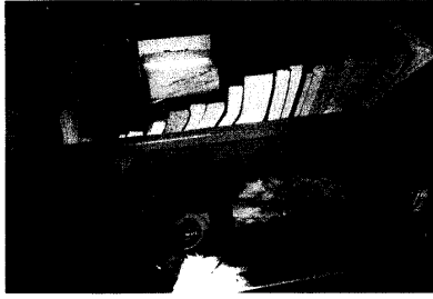
Boxes in loft compacting loft insulation reducing efficiency
