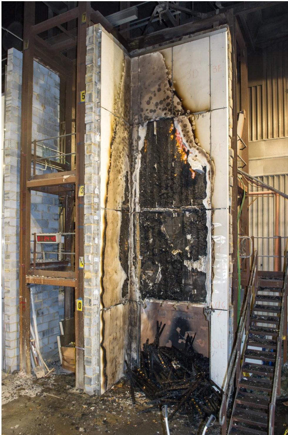
Figure 22. Full height photograph of system post-test – general.
