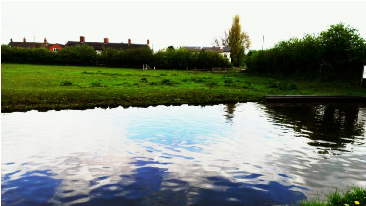
Location P4 – Looking East opposite Pasturefields Salt Marsh. Illustrates the fact that the canal is not elevated from the East and any surface-water contributions will be intercepted by the canal and conveyed to controlled canal overflow points. As such, the canal forms an effective barrier to surface-water flows from the East, with the exception of a few overflow points which drain into ditches.
