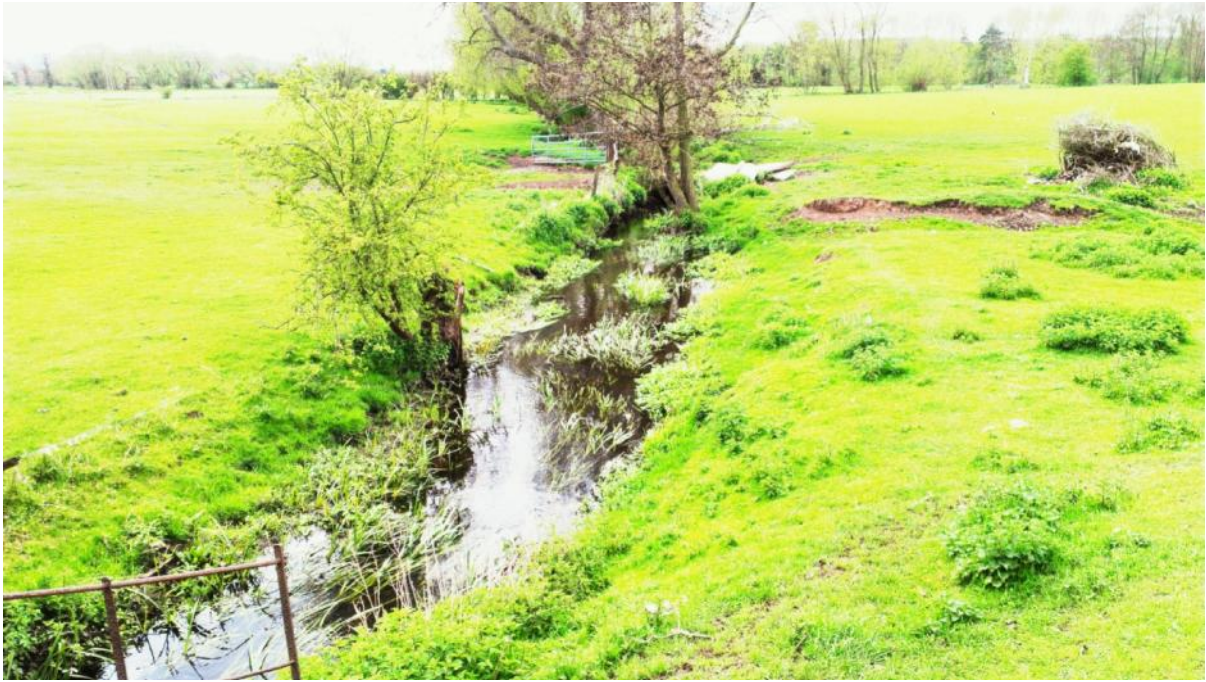
Location P3 – Looking West, brook crossing under canal and railway.
