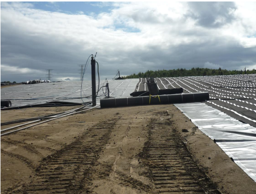
Capping layers (September 2017)
