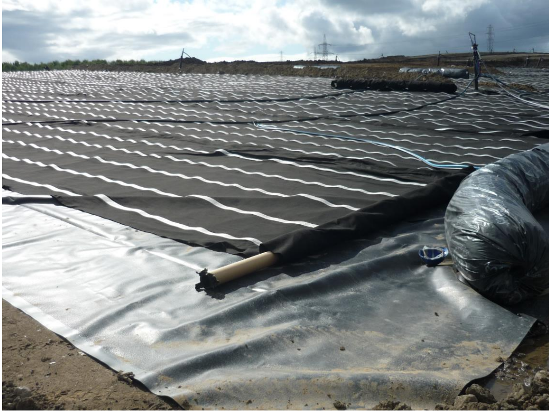
Capping layers (September 2017)
