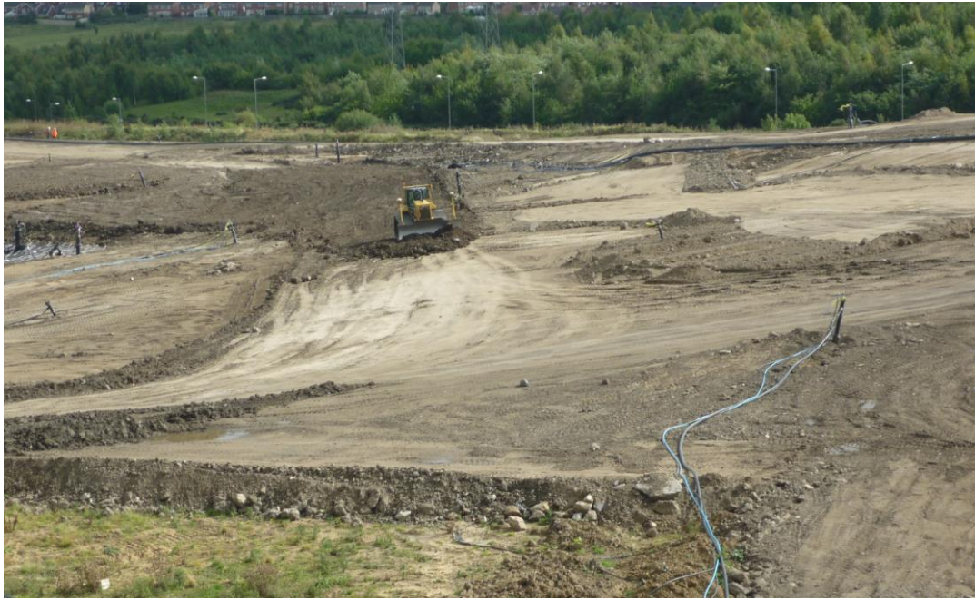
Placement of restoration soils (September 2017)
