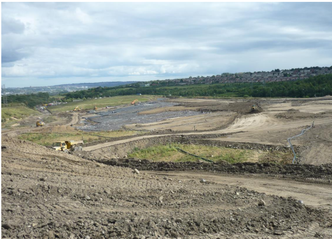
Whole site works (September 2017)
