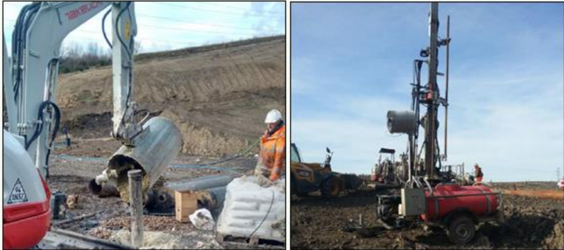
Gas well drilling works (March 2017)
