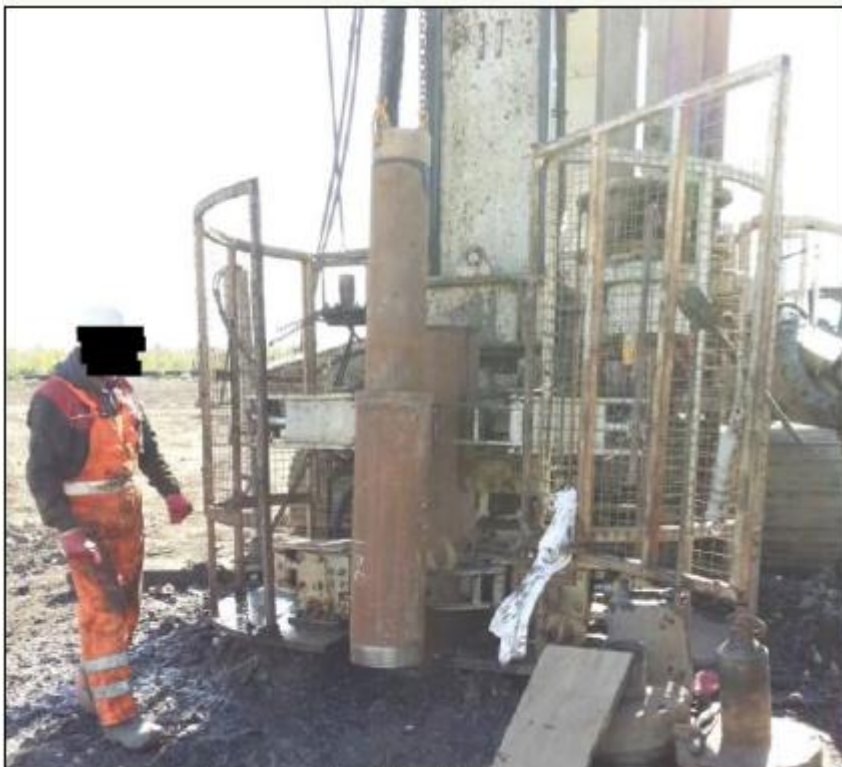
Leachate well works (April 2017)
