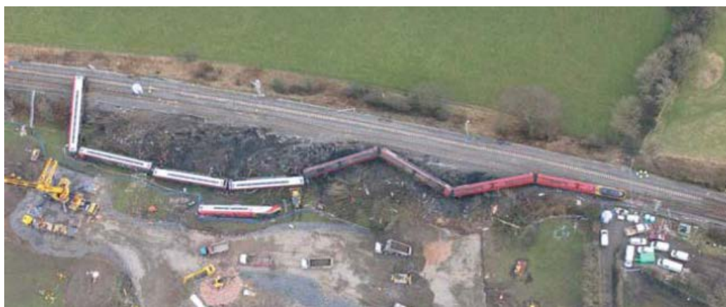
Figure 6: Derailment at Grayrigg
