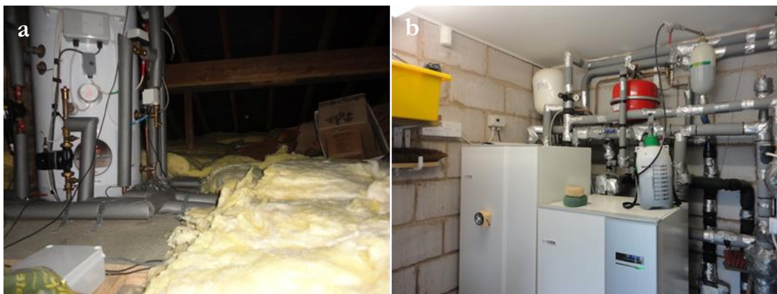
Figure 4-6. (a) Buffer tank (with additional bubblewrap to act as insulation) and circulation pumps in unheated shed (CS20), (b) location of the shed, to the right of blue door (CS20)
