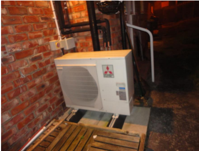
Figure 5-3. CS07 – External fan unit and installation
