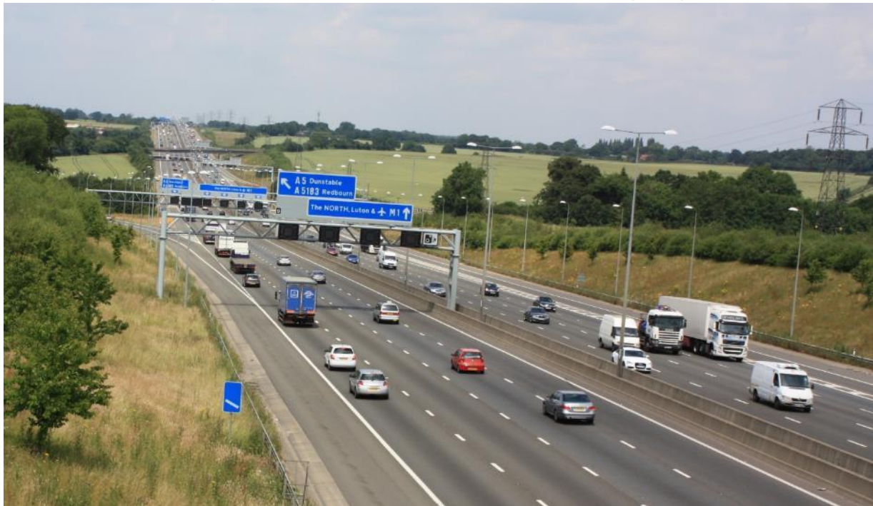
Figure 3.5 – Example of CCTV Cameras and Lighting
