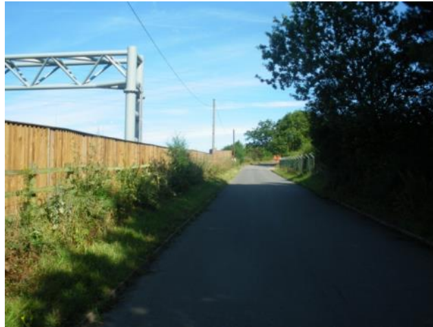
1 year after: noise barrier reduces view of traffic, gantry clearly visible.
