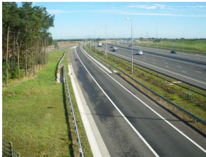
1 year after: considerable screening vegetation lost, noise barrier/screen installed.
