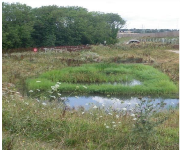
OYA: Well vegetated balancing pond close to Hempstead Road
