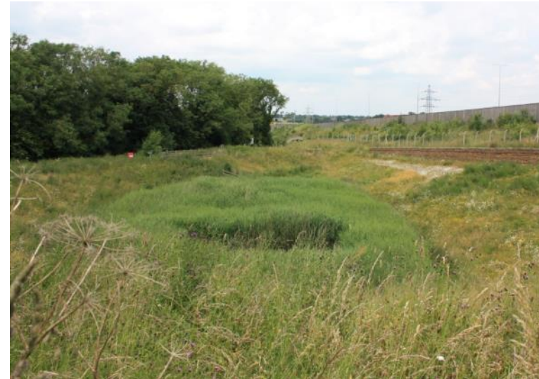
FYA: Well-maintained planting near Norringtonend Farm overbridge (OYA)
