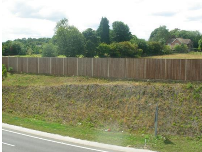
1 year after: considerable mature screening vegetation lost, noise barriers installed.
