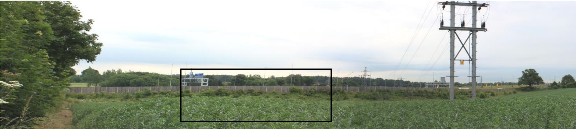
FYA: Gantry and lighting remain visible at FYA. Planting is progressing well.
