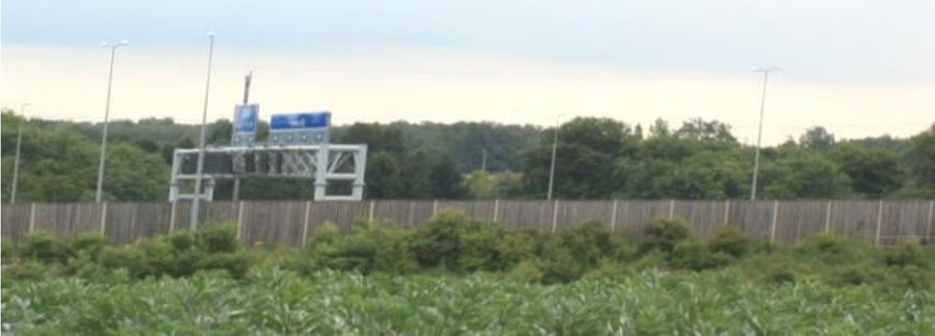
FYA - close up view of progress of planting adjacent to the environmental barrier
