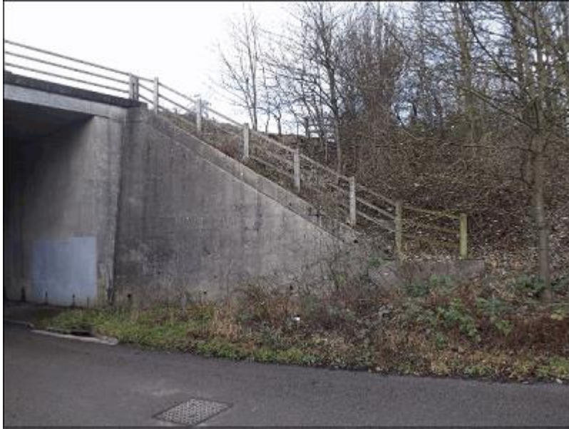
05 - North East Wing Wall 20.1.14
