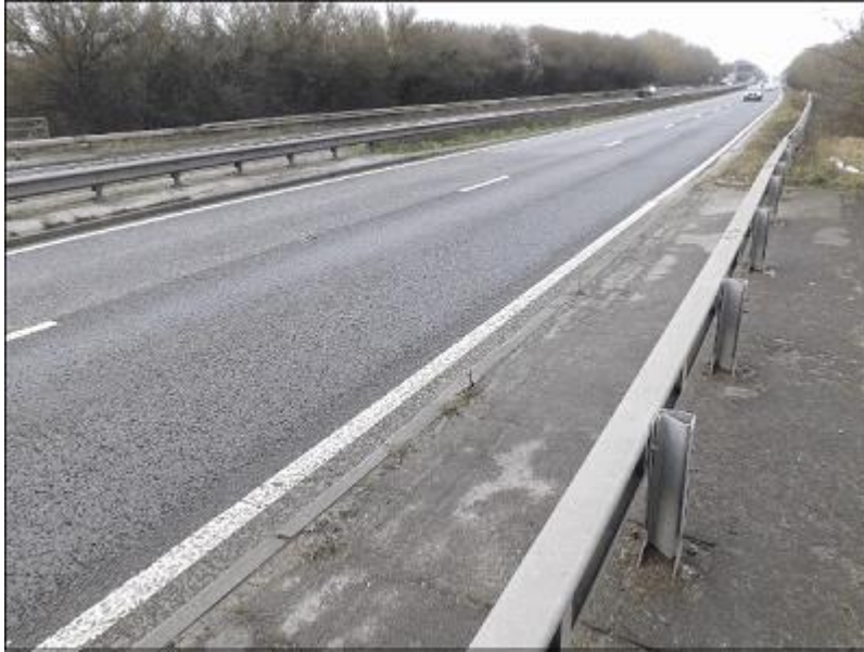
13 - View Over Southbound Carriageway Looking North 20.1.14
