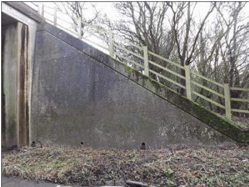
08 - South West Wing Wall 20.1.14
