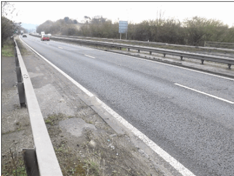
12 - View Over Southbound Carriageway Looking South 20.1.14
