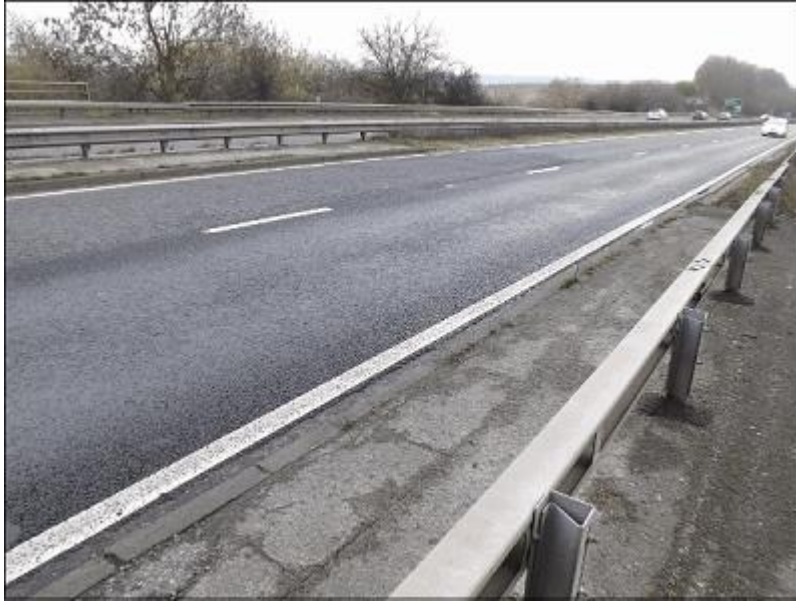
11 - View Over Northbound Carriageway Looking South 20.1.14
