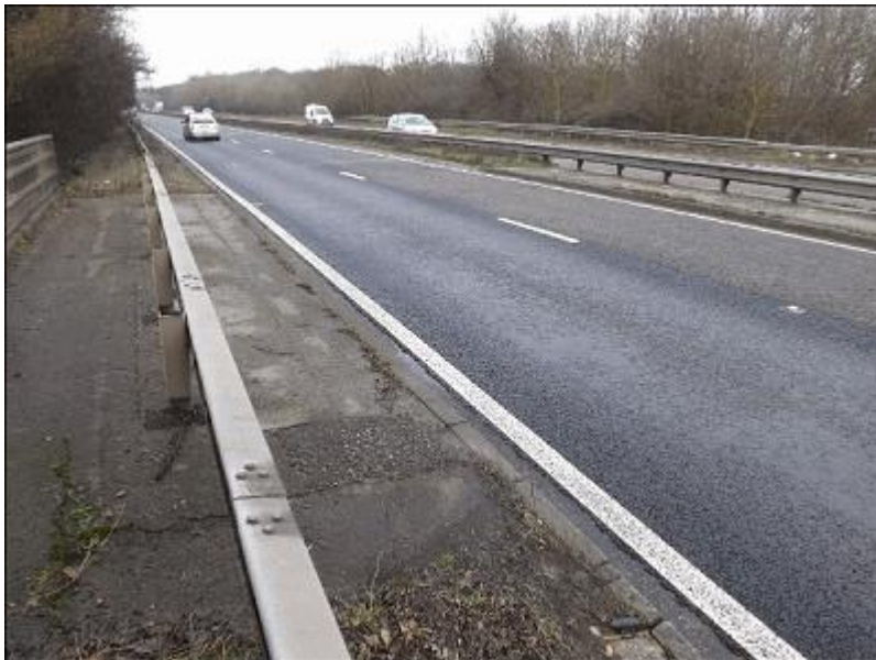
10 - View Over Northbound Carriageway Looking North 20.1.14
