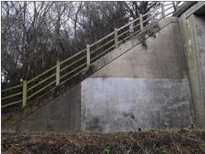
06 - North West Wing Wall 20.1.14
