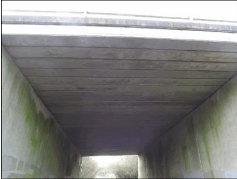
09 - Deck Soffit Looking West 20.1.14
