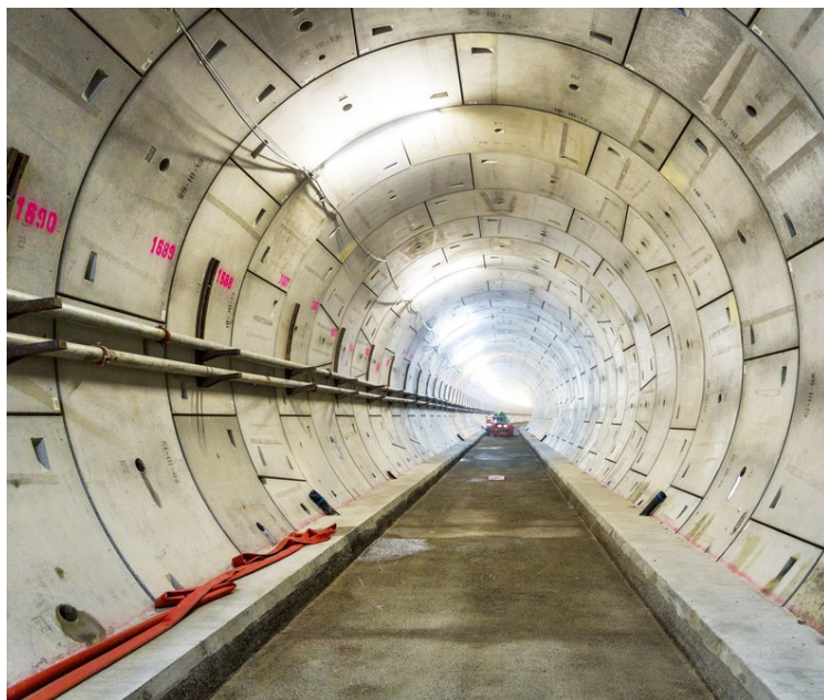
New rail tunnel, under construction for the London Crossrail Project.
